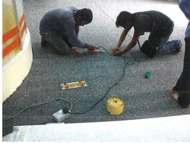
Picture 3.11 Installation of new carpet
