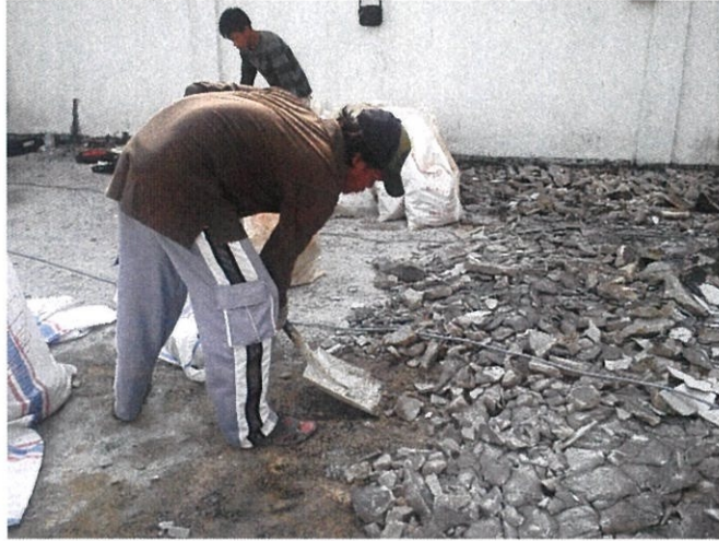
Picture 3.5 Cleaning work
