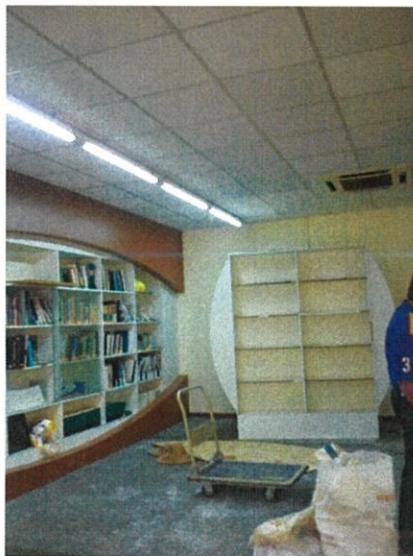
Picture 3.10 New suspended ceiling (gypsum mineral fibre)
