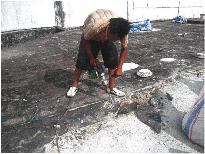
Picture 3.4 Drilling work to remove previous concrete layer
