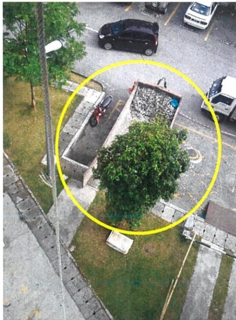
Picture 3.6 Trash container to remove the entire drilled concrete layer
