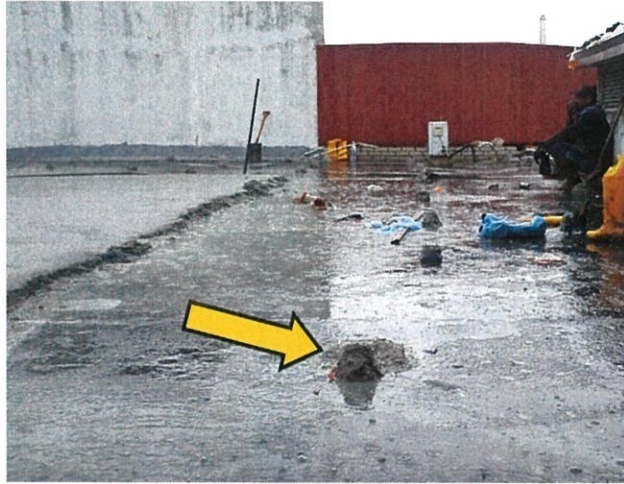
Picture 3.7 Leveling new concrete layer
