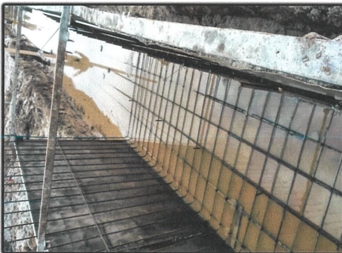
Photo 3.11: installation of reinforced drains, sabak bernam Selangor
