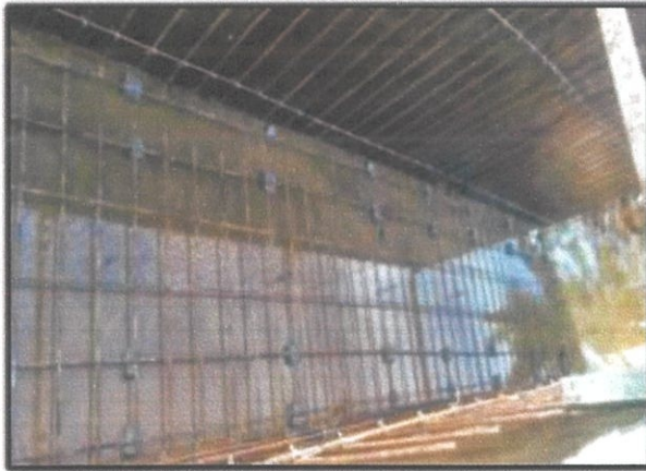
Photo 3.12: reinforced for floor drain, Sabak Bernam Selangor
