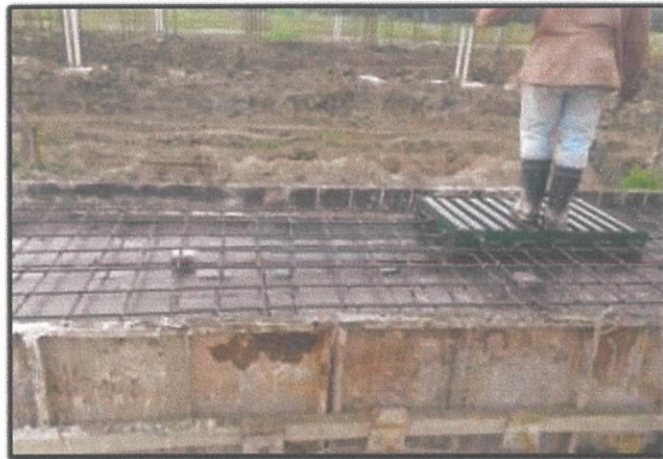
Photo 3.15: reinforced in floor drain, sabak bernam selangor
