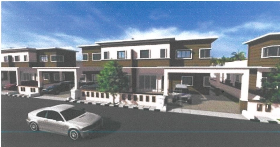
Photo 2.4: double storey, Sabak Bernam Selango
