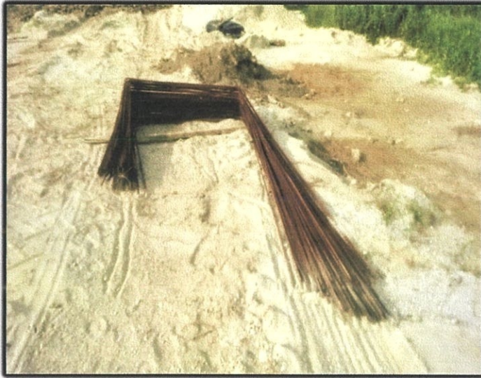
Photo 3.10: reinforced that has been bent for drains, sabak bernam selangor
