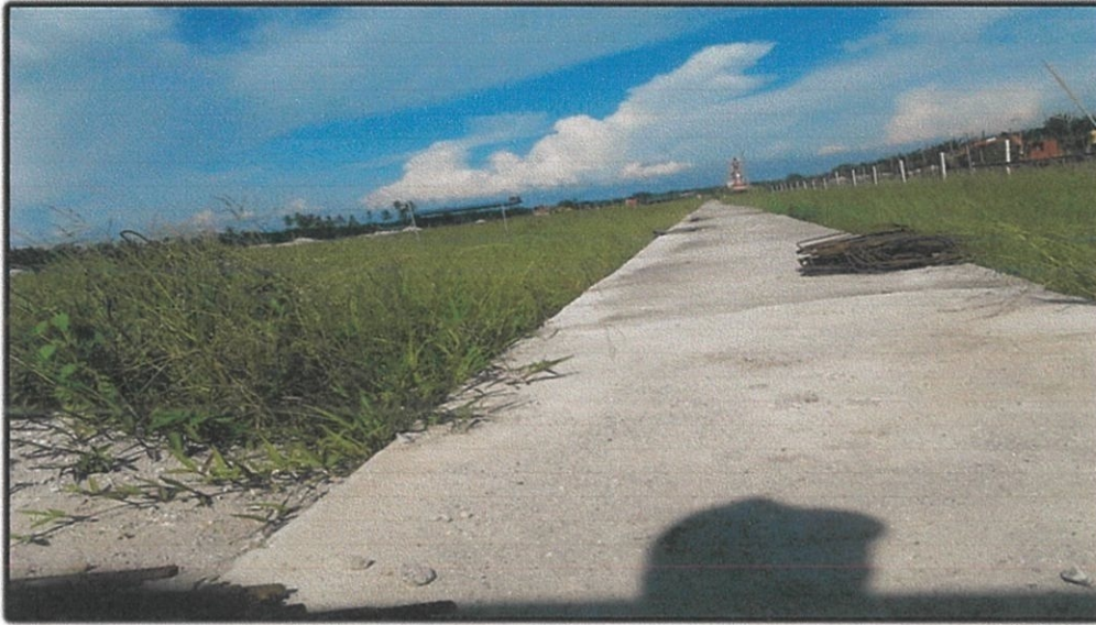
Photo 3.1: reinforced in-situ concrete drain.
