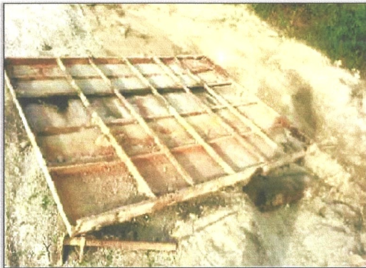
Photo 3.8: molds use to install the wall drains, sabak bernam selangor
