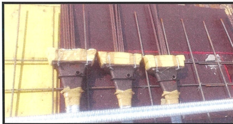
Photo 3.25 Anchorage device at stretching end
