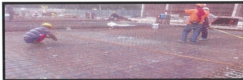
Photo 3.21 The general workers tie the bottom reinforcement bars
