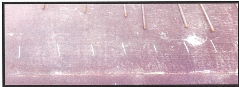
Photo 3.20 The spacing between reinforcement bars was marked by using a chalk
