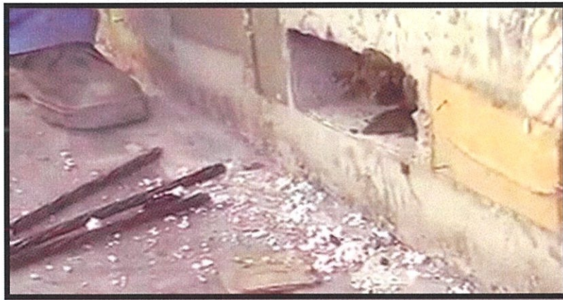
Photo 3.38 Extra strands being cut after the stressing process
