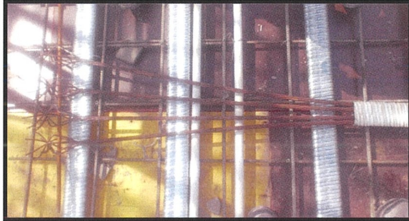
Photo 3.28 Anchorage device at dead end zone
