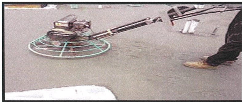
Photo 3.33 Troweling machine used to get good finish for slab
