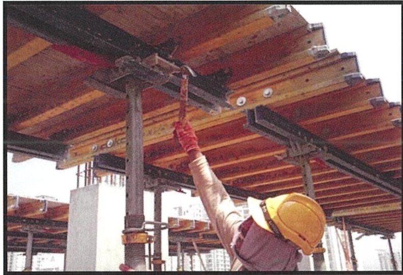
Photo 3.15 The worker tightens the swivel-head by using a hammer
