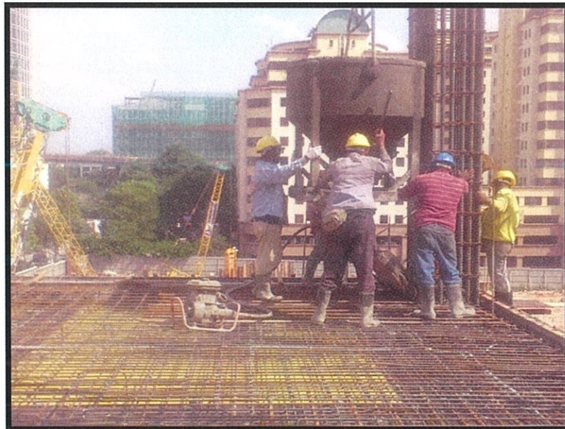
Photo 3.31 The workers concreting the slab from the corner area
