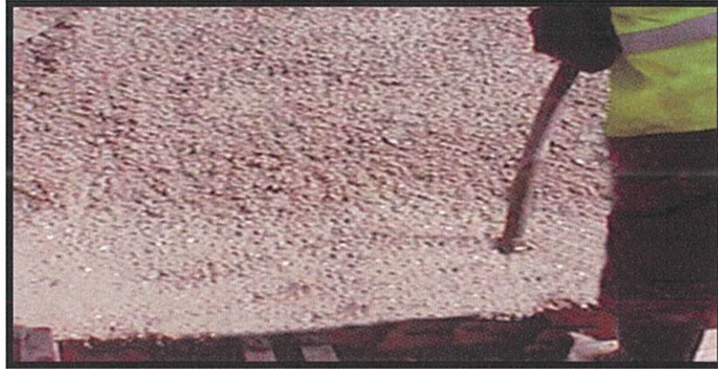
Photo 3.32 Concrete vibrator machine used to compact concrete
