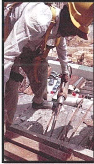
Photo 3.36 Mono jack machine connected to the first cable
