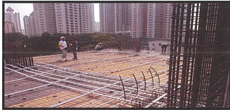
Photo 3.26 Installation of flat duct sheathings and strands
