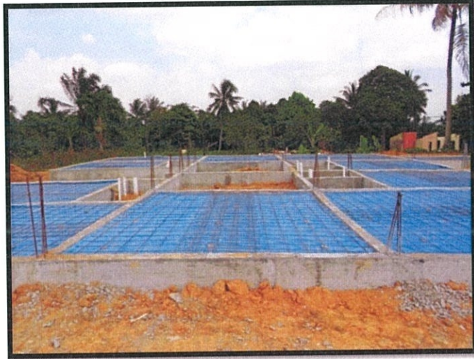
Figure 7: Reinforcement Bar at Floor Slab
