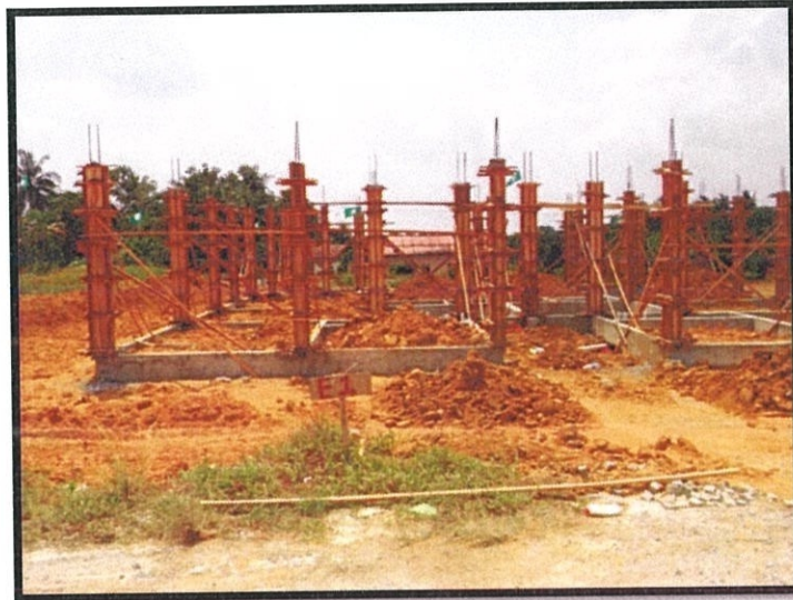
Figure 12: Formwork of column
