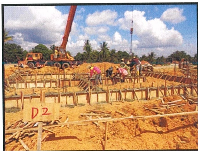
Figure 11: Formwork of Ground Beam
