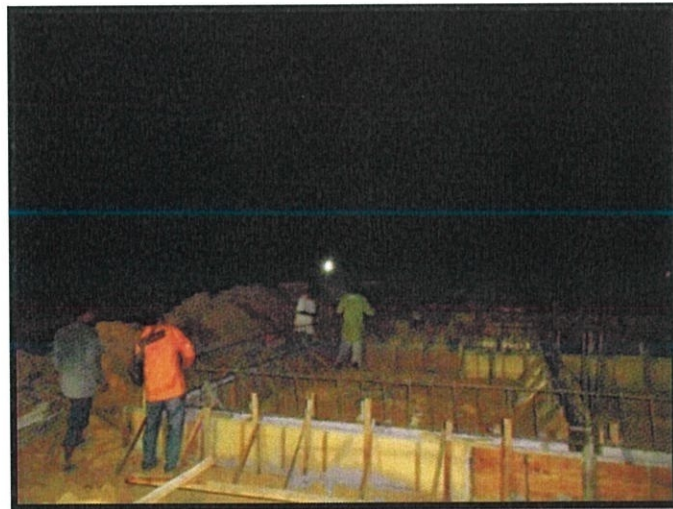
Figure 6: Reinforcement Bar at Ground Beam
