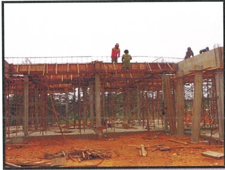
Figure 9: Reinforcement Bar at Roof Beam
