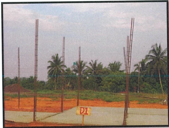
Figure 8: Reinforcement Bar at Column
