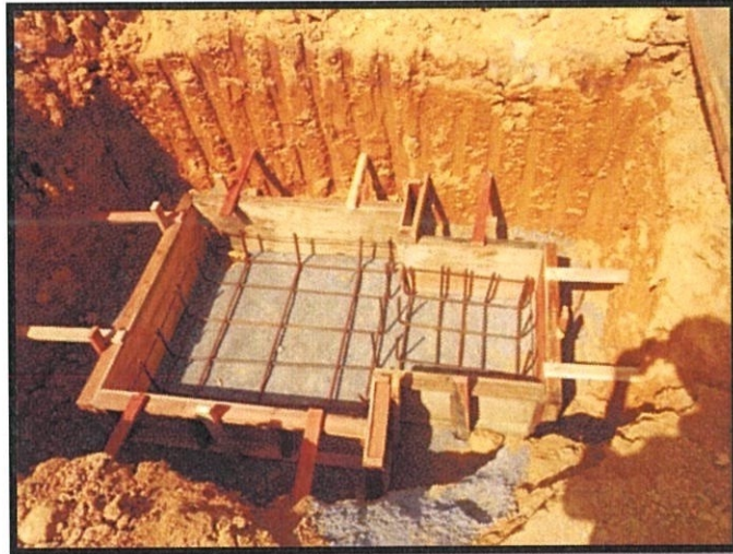
Figure 5: Reinforcement Bar at Footing
