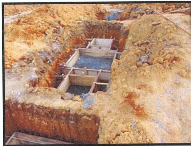
Figure 10: Formwork of Footing
