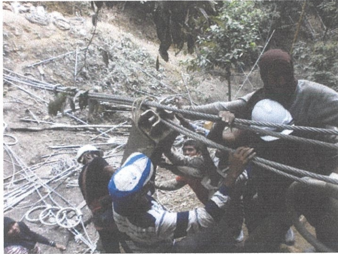
Appendix 7: Installation of post.
