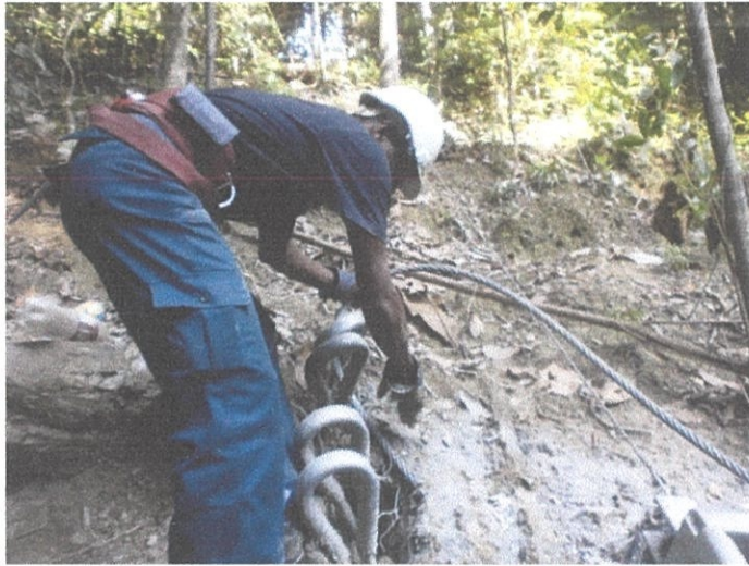
Appendix 6: Installation of support ropes
