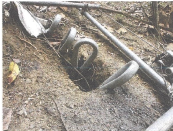
DIAGRAM 3.2.2.9 Arrangement of flexible heads
