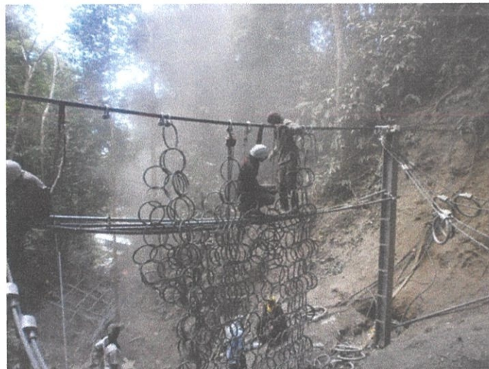
Appendix 8: Installation of ring net.
