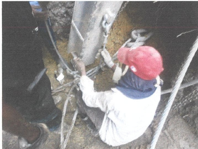
Appendix 10: Installation of overturn securing ropes
