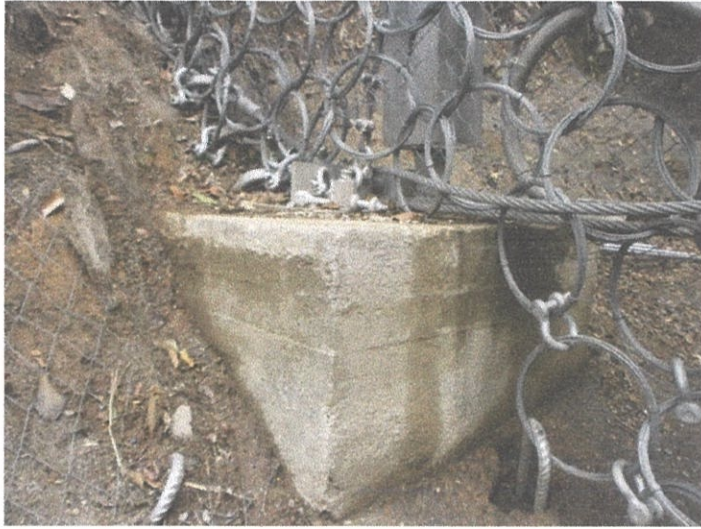
Appendix 3: Post foundation.
