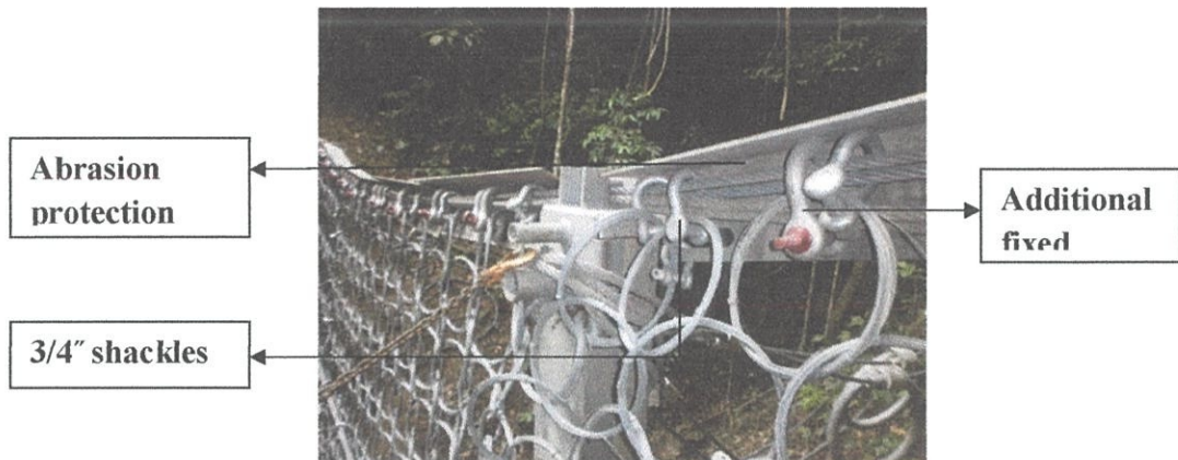
DIAGRAM 3.2.3.11 Additional fixed shackles to avoid torsion.
