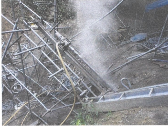
Appendix 1: Drilling work.
