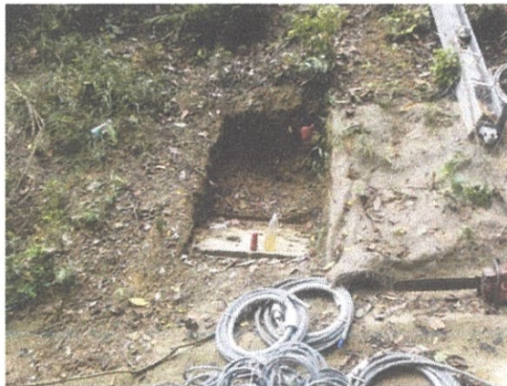
DIAGRAM 3.2.2.4 Post foundation
