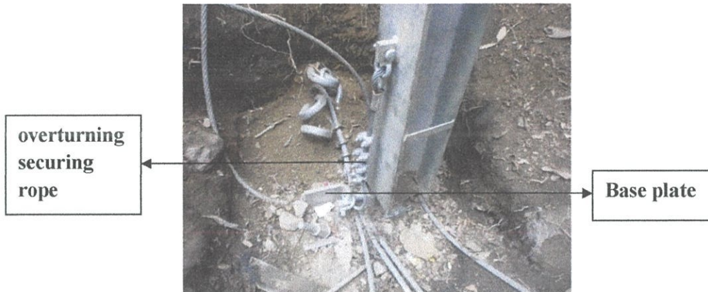
DIAGRAM 3.2.3.2 Overturn securing rope
