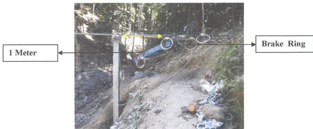
DIAGRAM 3.2.3.5 Brake rings should be 1 meter away from the post
