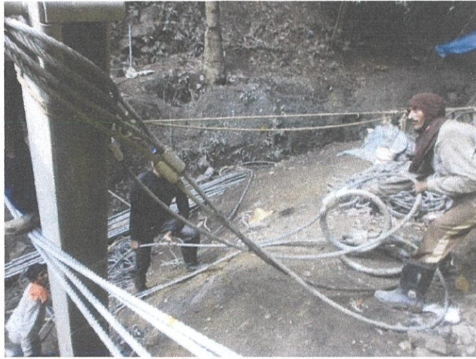
Appendix 9: Installation of flexible ropes.
