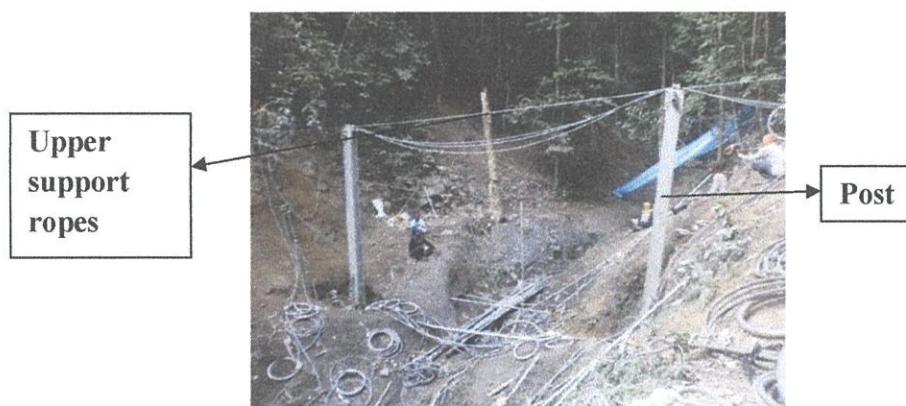
DIAGRAM 3.2.3.1 Upper support ropes
