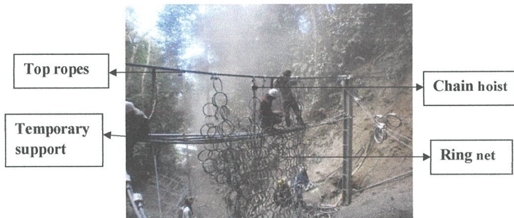
DIAGRAM 3.2.3.6 Alternatively a staging as a temporary support
