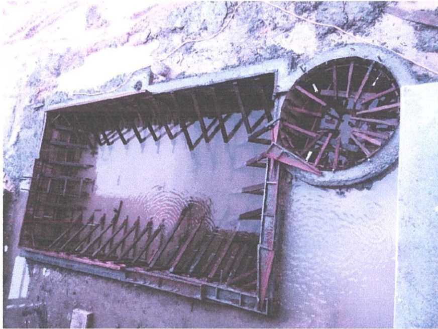
Photo 3.19: Cementing work in swimming pool
