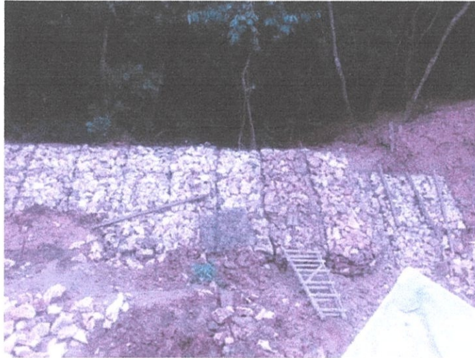
Photo 3.13: Layer of gabion wall
