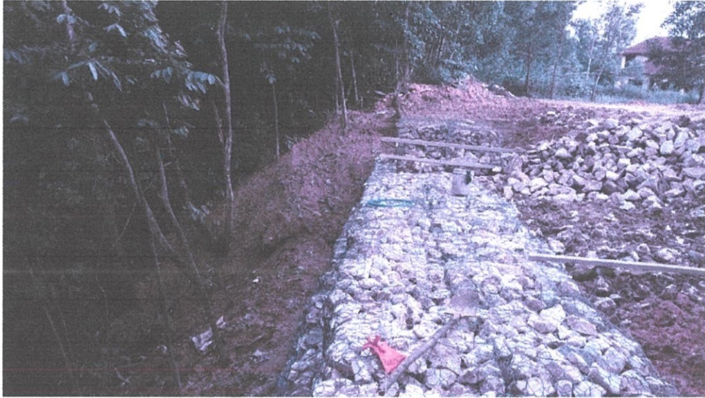
Photo 3.12: Arrange of gabion wall
