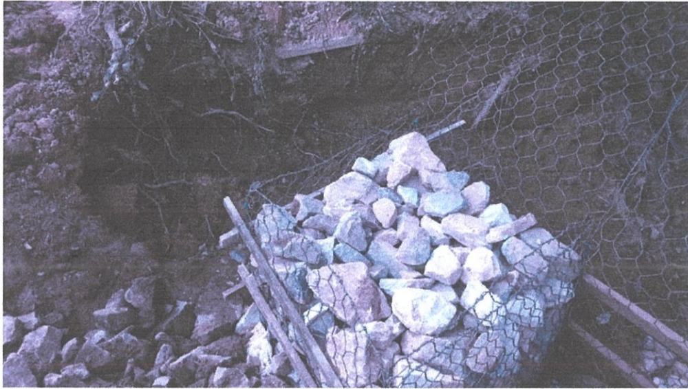
Photo 3.10: Arrangement of stones in basket gabion wall
