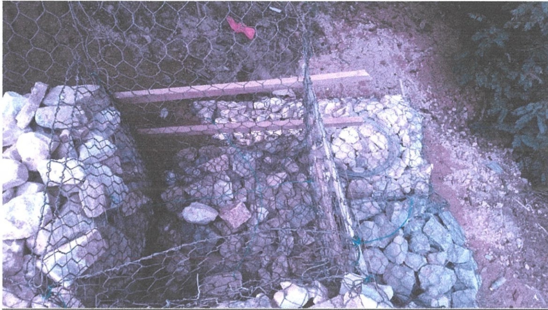
Figure 3.8: Gabion Installation Instruction
