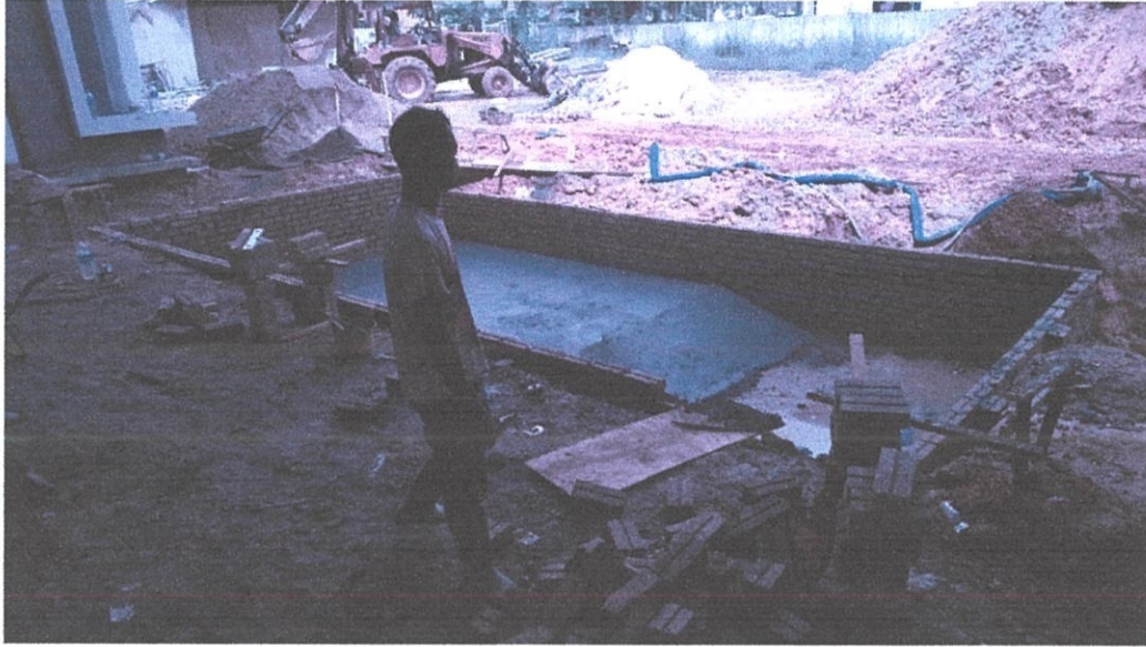
Photo 3.16: The binding brick work
