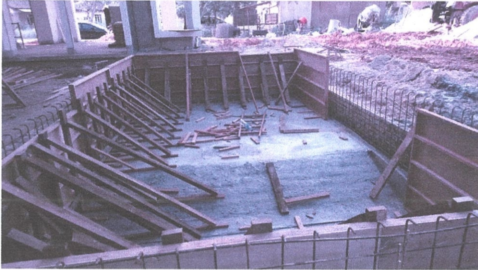
Photo 3.18: Installation of frame
