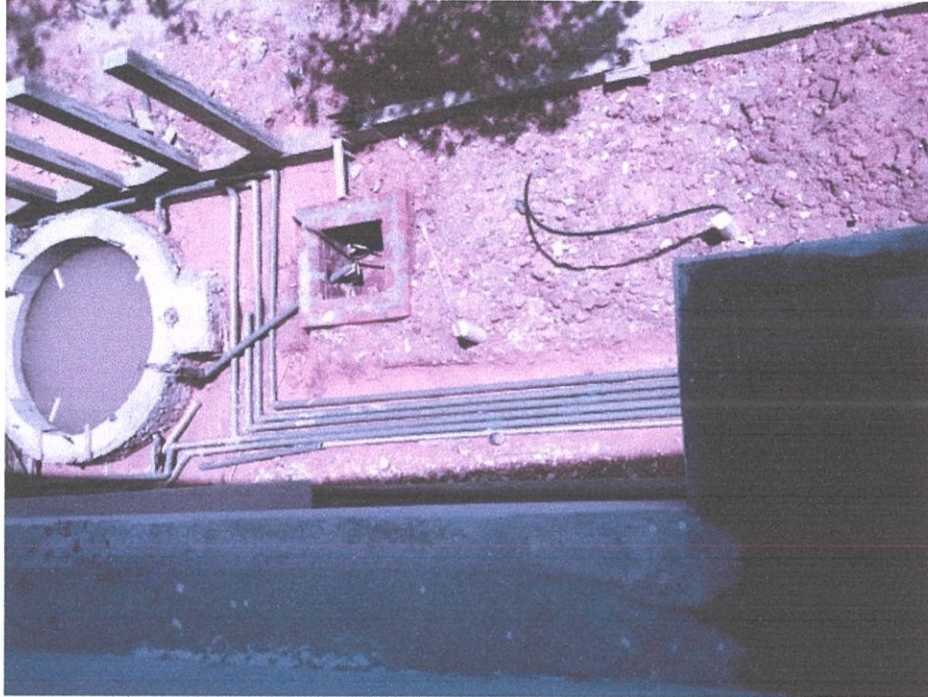
Photo 3.22: Installation of piping swimming pool
