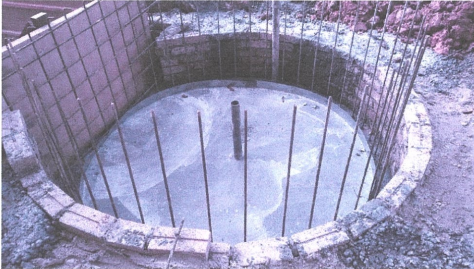
Photo 3.17: Installation of framework steel
