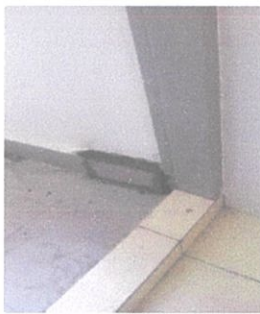
Picture 3.23: Worker fill up the cement at grid line
