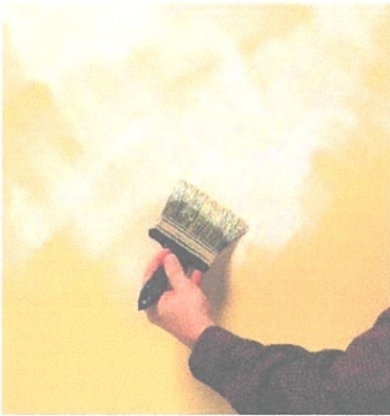
Picture 3.13: Paint the wall
