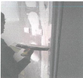
Picture 3.7: The worker put the skim coat
