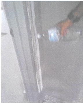
Picture 3.6: The workers have pour the water on the wall
