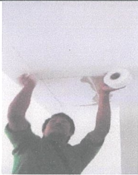
Picture 3.17: Use fiberglass tape to the ceiling
