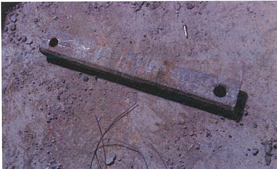
Photo 3.29: Deck Beam Bar
