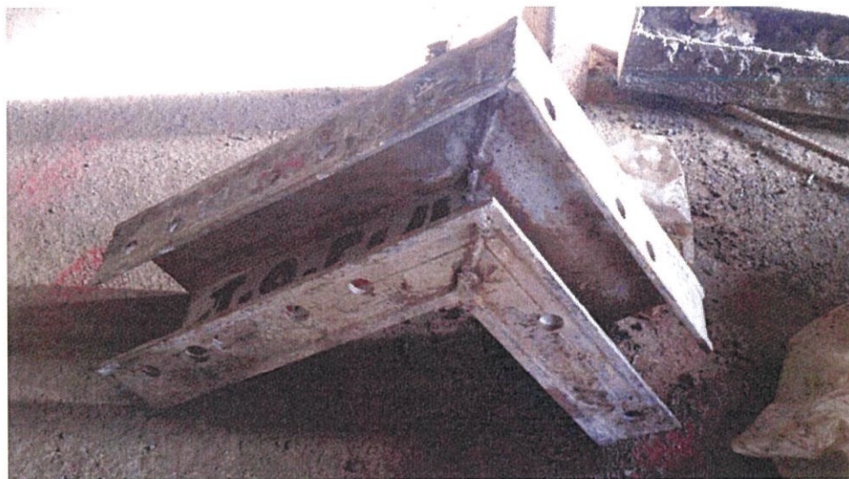
Photo 3.35: External Soffit Corner
