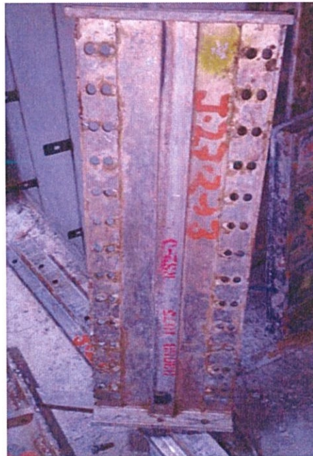
Photo 3.16: Beam Soffit Bulkhead
