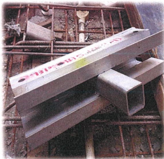
Photo 3.14: Prop Head for Soffit Beam
