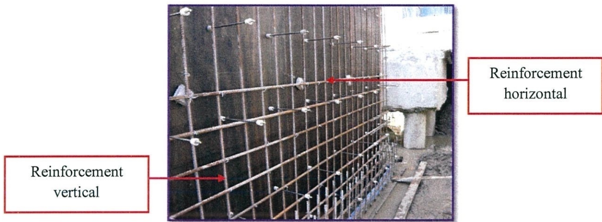
Photo 4.27: The installation reinforcement wall in STP
