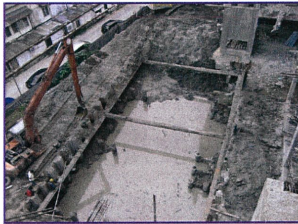
Photo 4.9: The excavation works for the construction of STP
