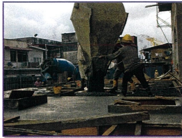
Photo 4.42: Concreting work for top slab use the grade concrete 35
