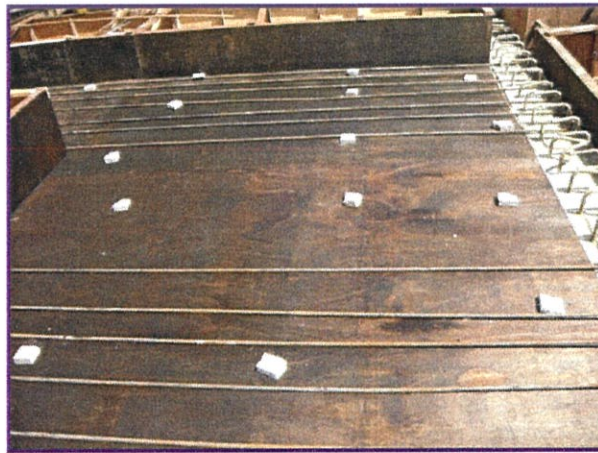
Photo 4.39: Spacing block will put before install reinforcement
