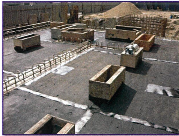
Photo 4.37: The installation opening formwork on top slab
