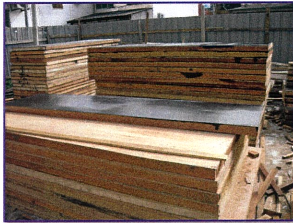
Photo 4.12: Black oil will use on surface of formworks
