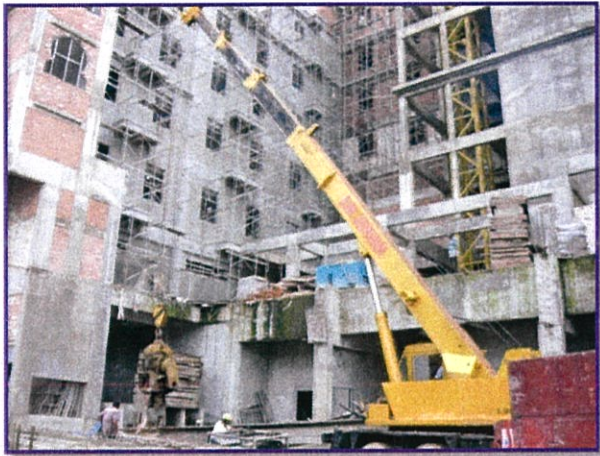
Photo 4.7: Mobile crane used to lifted vibrate hammer
