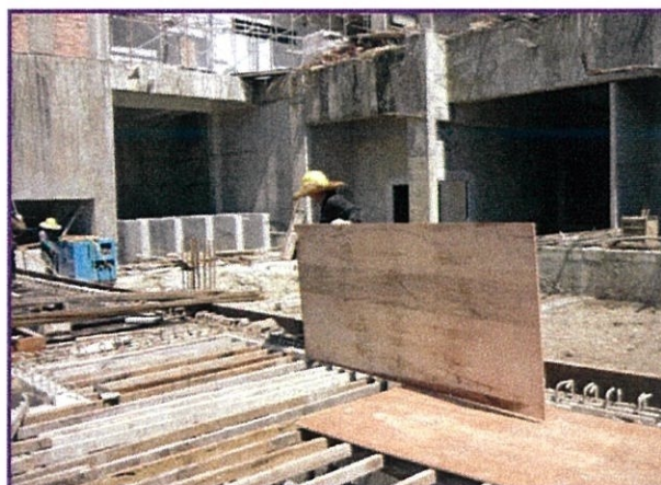
Photo 4.36: The installation plywood on top slab
