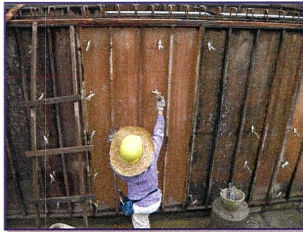
Photo 4.31: The installation external formwork wall in STP
