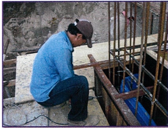
Photo 4.29: Water stop install to continue wall
