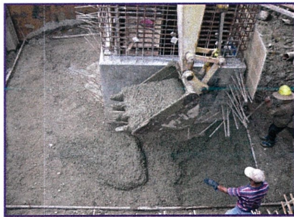
Photo 4.16: Lean concreting work in STP to do by the concreter
