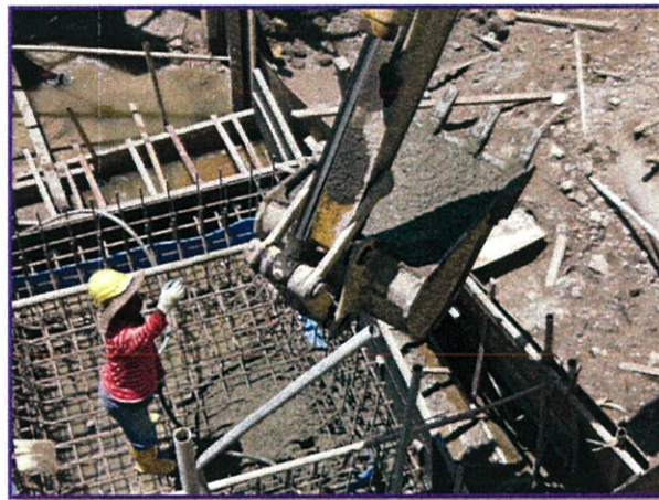
Photo 4.24: Concreting works for slab in STP
