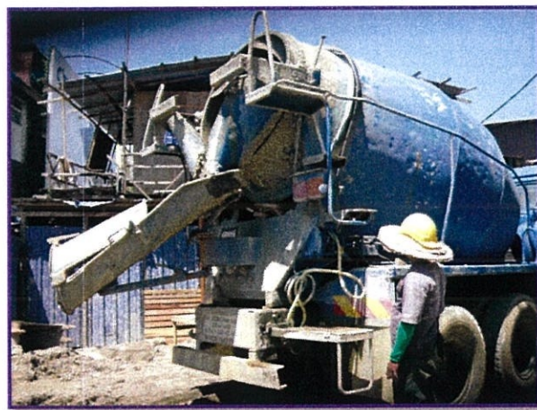
Photo 4.23: Ready mix concrete
