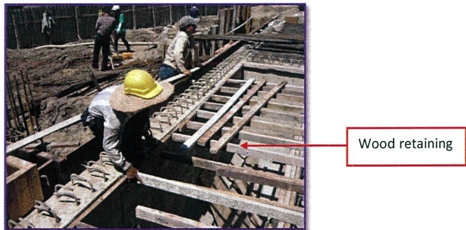
Photo 4.35: The installation wood retaining size in STP
