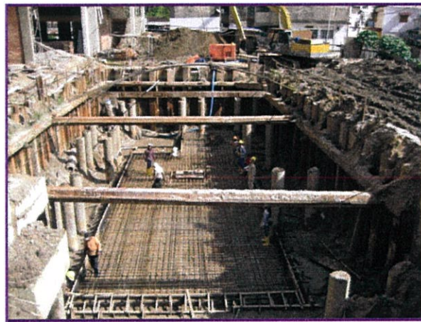
Photo 4.18: The installation of reinforcement slab for STP
