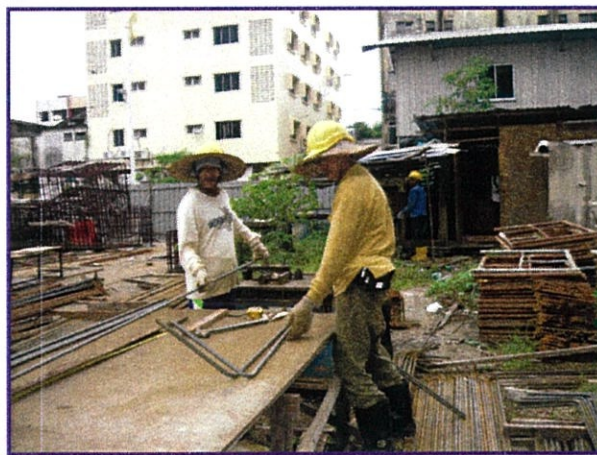
Photo 4.17: The bending reinforcement doing by the bar benders
