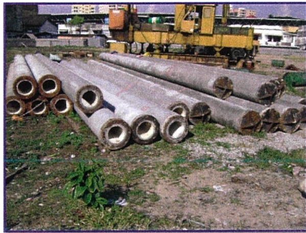
Photo 4.1: Spun pile with diameter 450 mm to support loading
