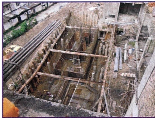
Photo 4.26: The installation of reinforcement for wall STP
