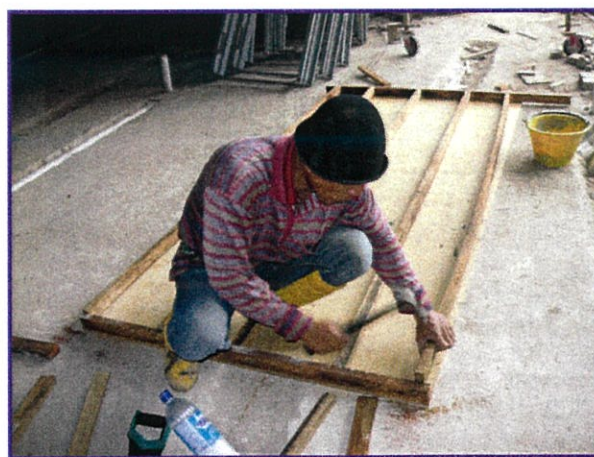
Photo 4.11: The carpenter do formworks follow the measurement
