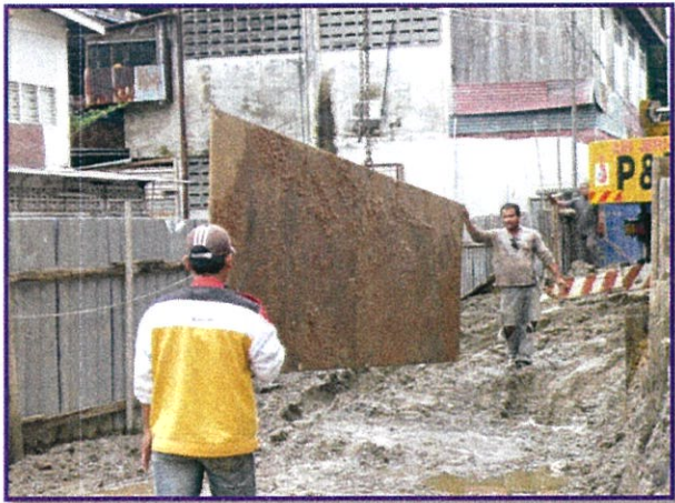
Photo 4.6: The sheet plate lifted by the mobile crane
