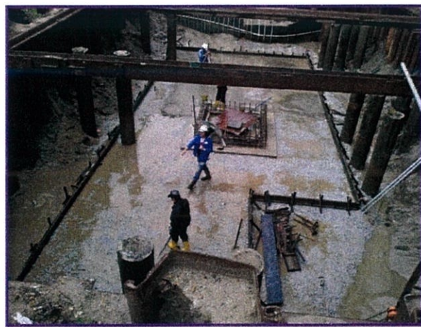
Photo 4.15: The size crusher run used is 1-1/2" and compact in STP.
