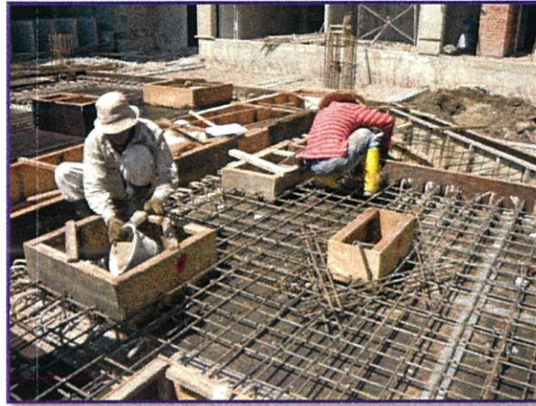
Photo 4.40: The installation reinforcement to do by the bar bender
