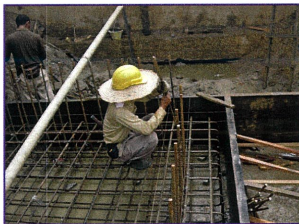
Photo 4.19: The installation of reinforcement for wall
