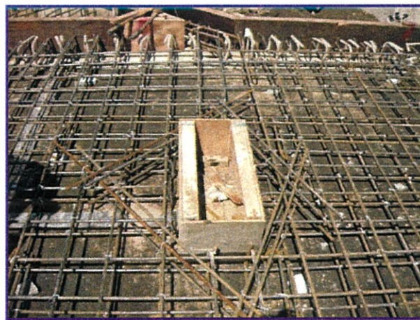
Photo 4.41: The installation reinforcement for opening
