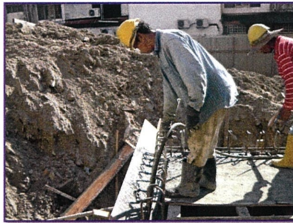
Photo 4.33: Vibration works to concreting
