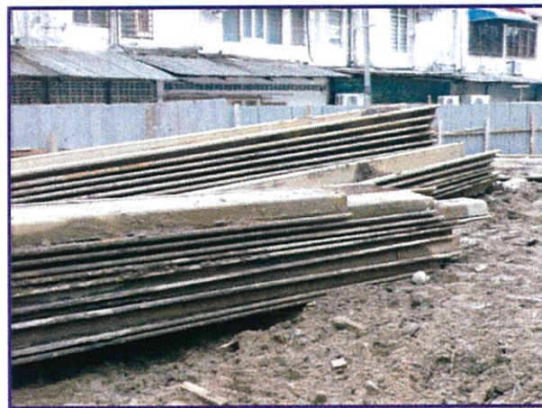
Photo 4.3: The length Steel sheet piles used is six (6) meter
