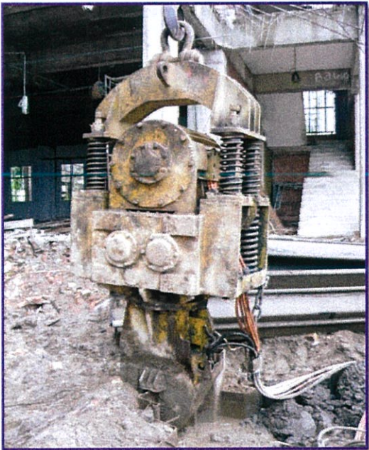
Photo 4.8: Vibrate hammer used to vibration to steel sheet piles
