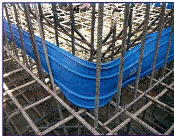
Photo 4.30: Water stop install in slab below STP.
