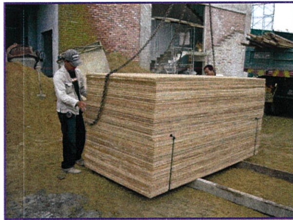
Photo 4.10: Site supervisor checking the plywood arrived in site
