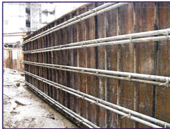
Photo 4.32: The cellular steel used as retaining formworks
