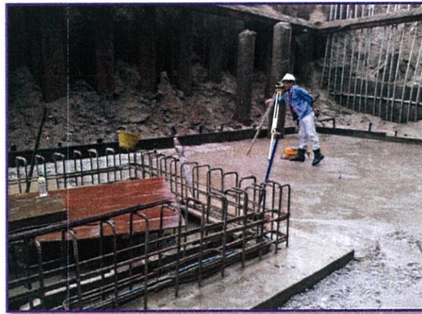
Photo 4.2: Setting out, level and measurement by the Land Surveyor
