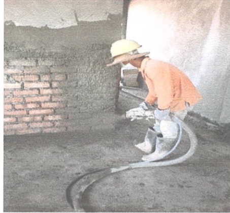
Photo 3.3: Spray to prepared surface
