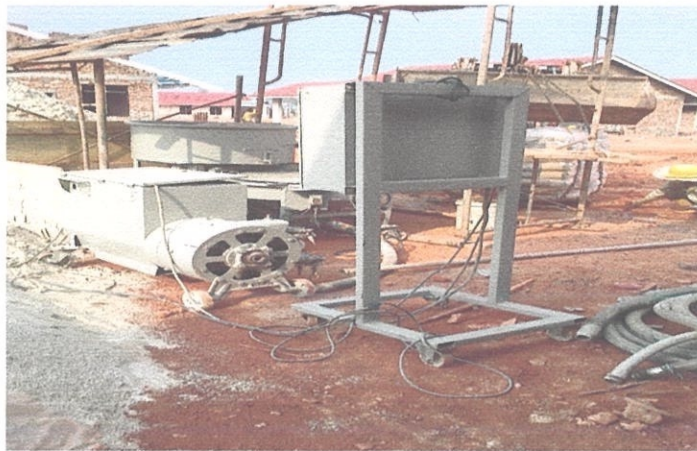
Photo 3.2: Mixture process placing
