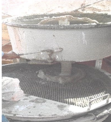
Photo 3.12: Separate any unwanted substances for plastering.
