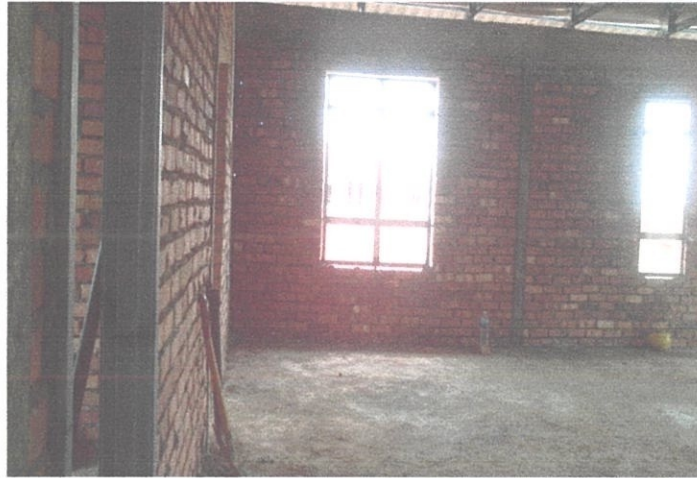
Photo 3.1: Surface Prepared For Plastering
