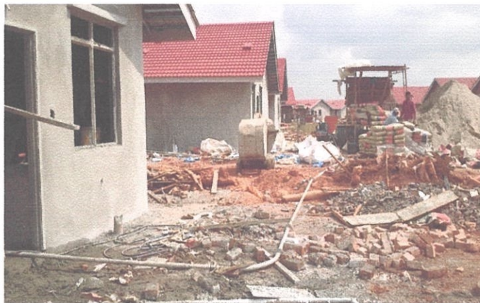
Photo 3.13: Plastering work started
