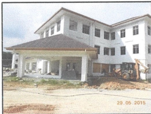
Photo 3.6: View of administration block
