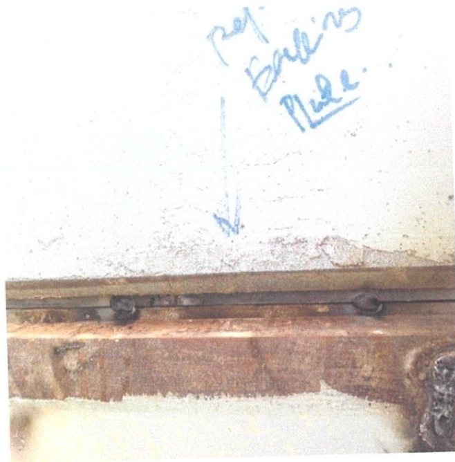
Photo 3.17 Backing plate repair
