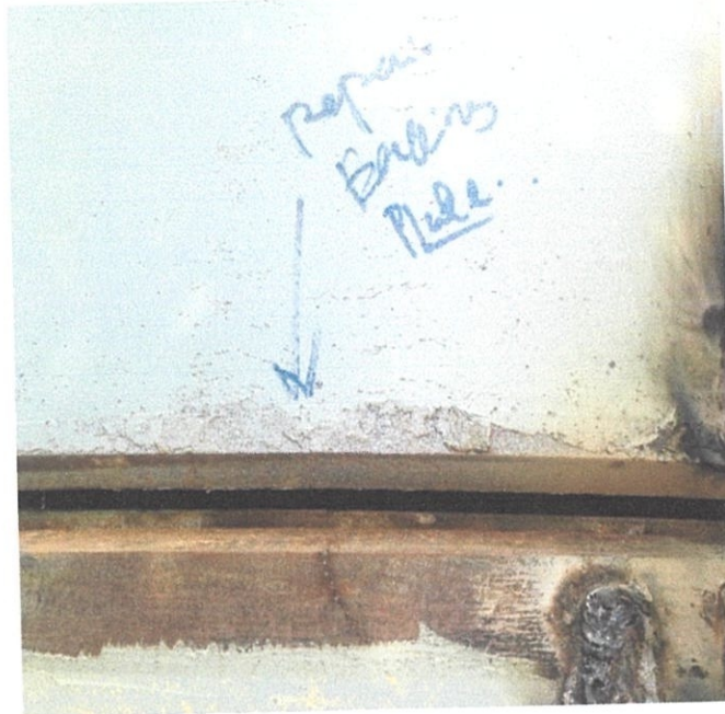
Photo 3.16 Backing plate repair
