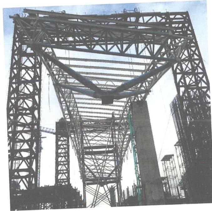
Photo 3.13 Jacking of main truss
