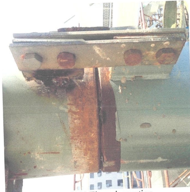
Photo 3.10 Fit-up inspection
