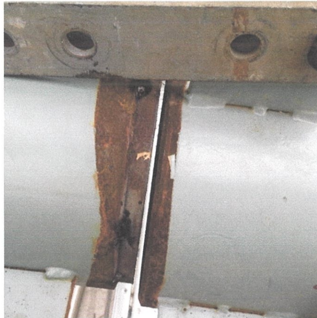
Photo 3.18 High and low jointing
