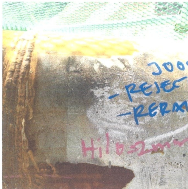
Photo 3.14 Welding spatter
