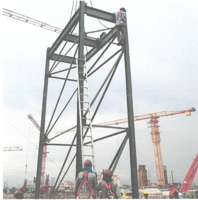
Photo 3.2 Temporary JIG support
