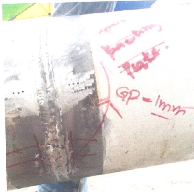
Photo 3.15 Welding spatter removal
