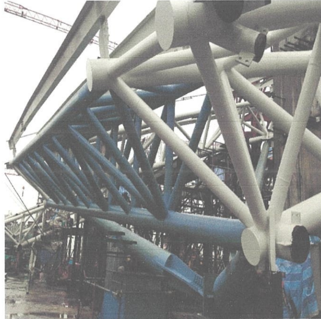
Photo 3.7 Eaves truss
