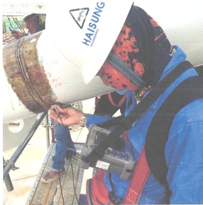
Photo 3.12 Ultrasonic inspection (UT)
