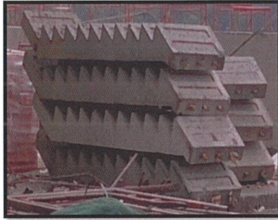
Photo 3.6 Stack of staircase after dismantle
