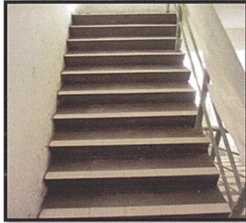
Photo 3.13 Finished of staircase
