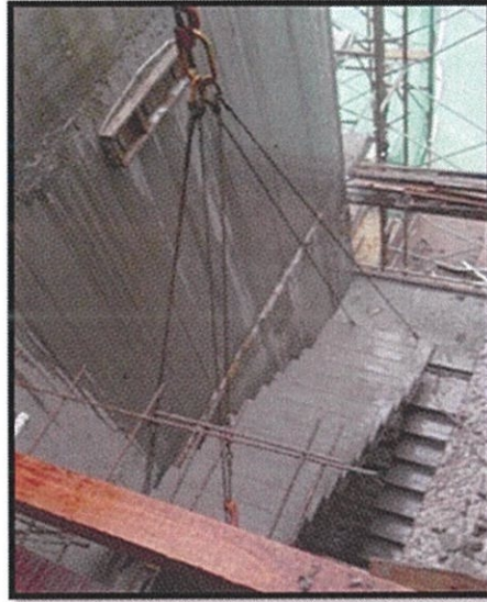
Photo 3.7 Lifting the staircase
