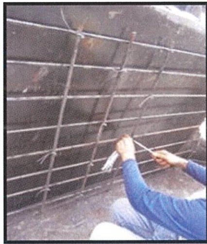
Photo 3.3 Forming of reinforcement bar
