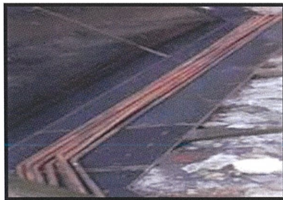
Photo 3.15 Reinforcement bar T12
