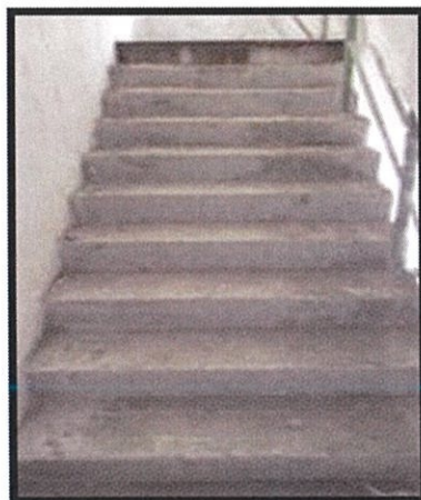
Photo 3.10 Complete installation of precast staircase
