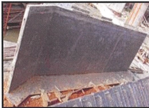
Photo 3.19 Base plate mould
