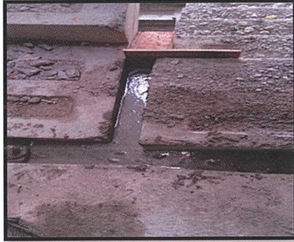
Photo 3.11 grouting the staircase
