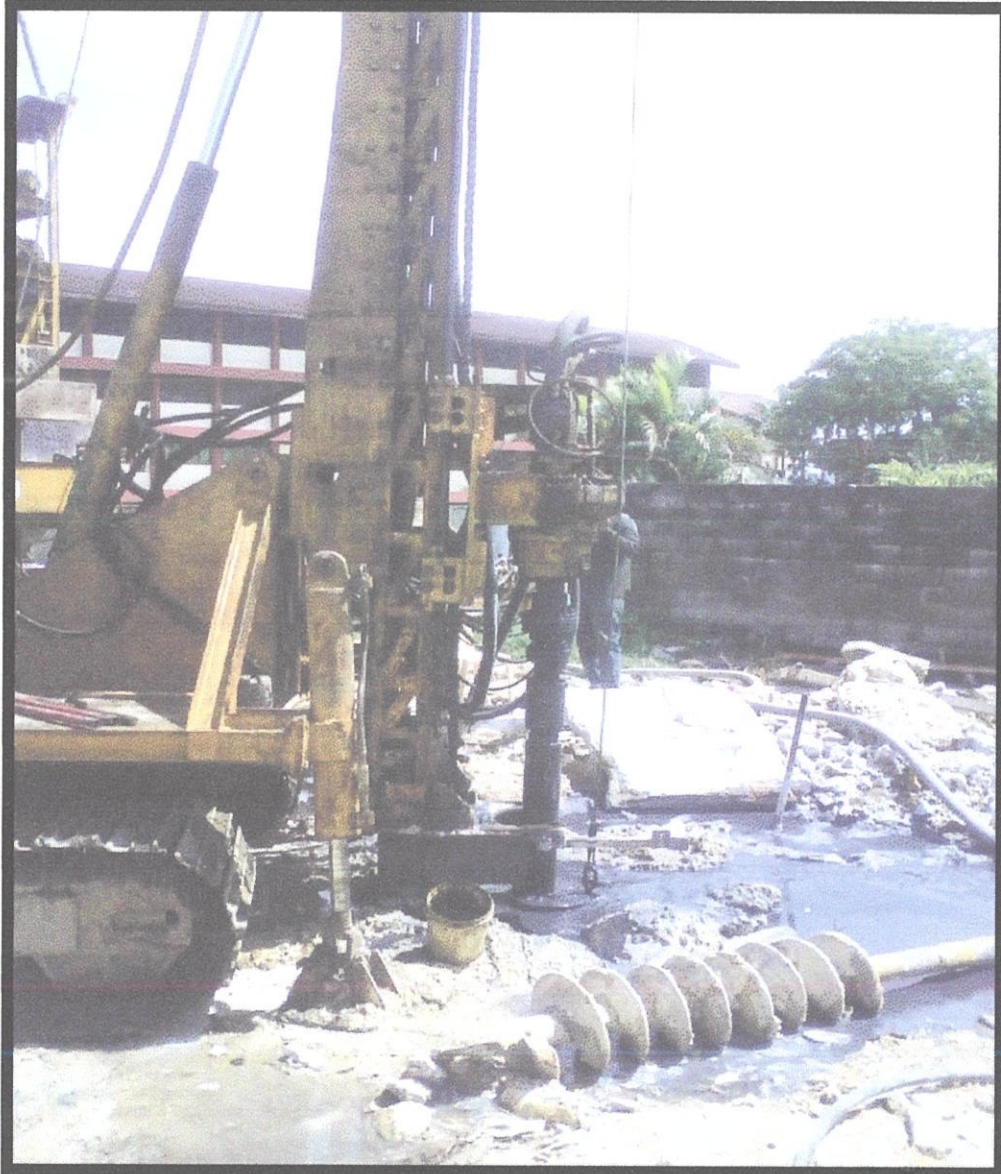
Gambarfoto 3.3 : Jentera 'Bore Piles'
