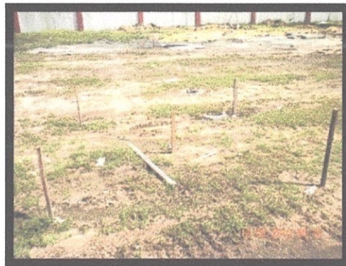
Gambarfoto 5.3 : kesilapan semasa 'marking' 'point'
