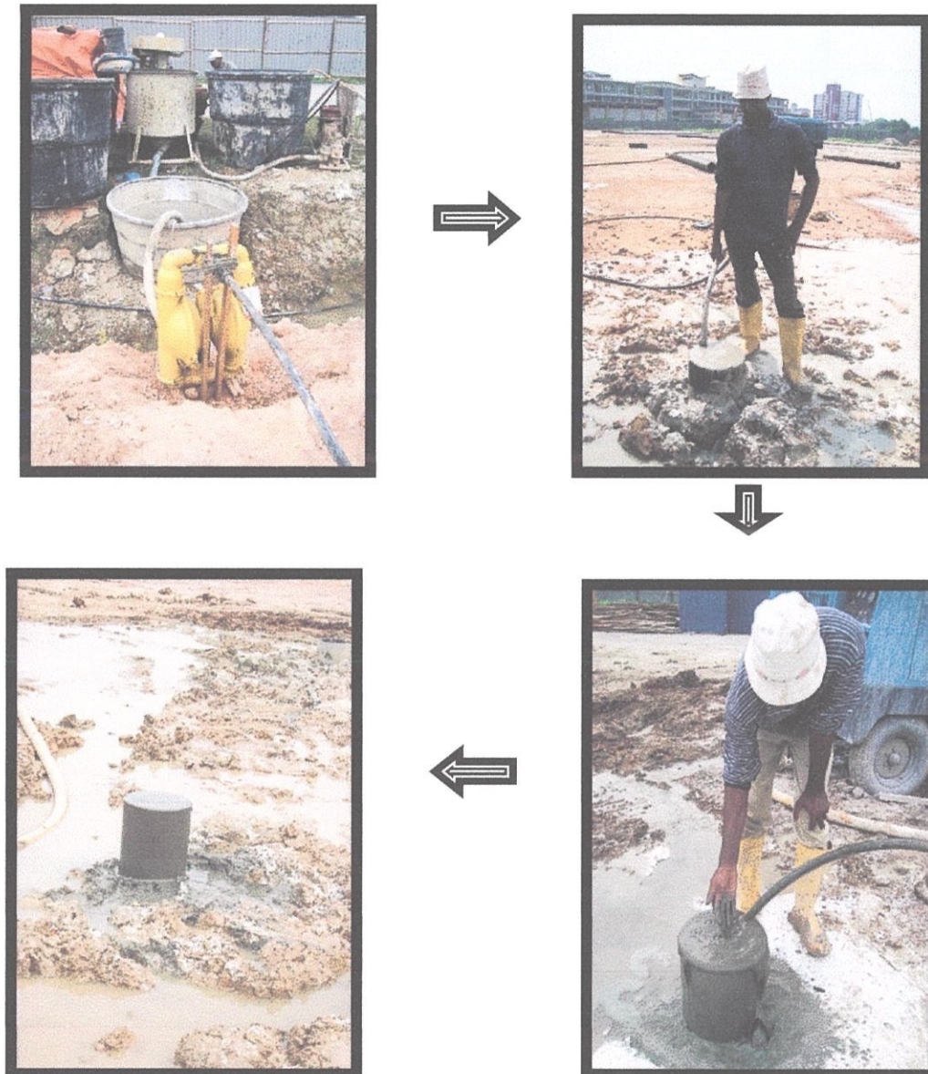
Gambarfoto 4.27 : Carta Proses Perekat (Grouting) 2
