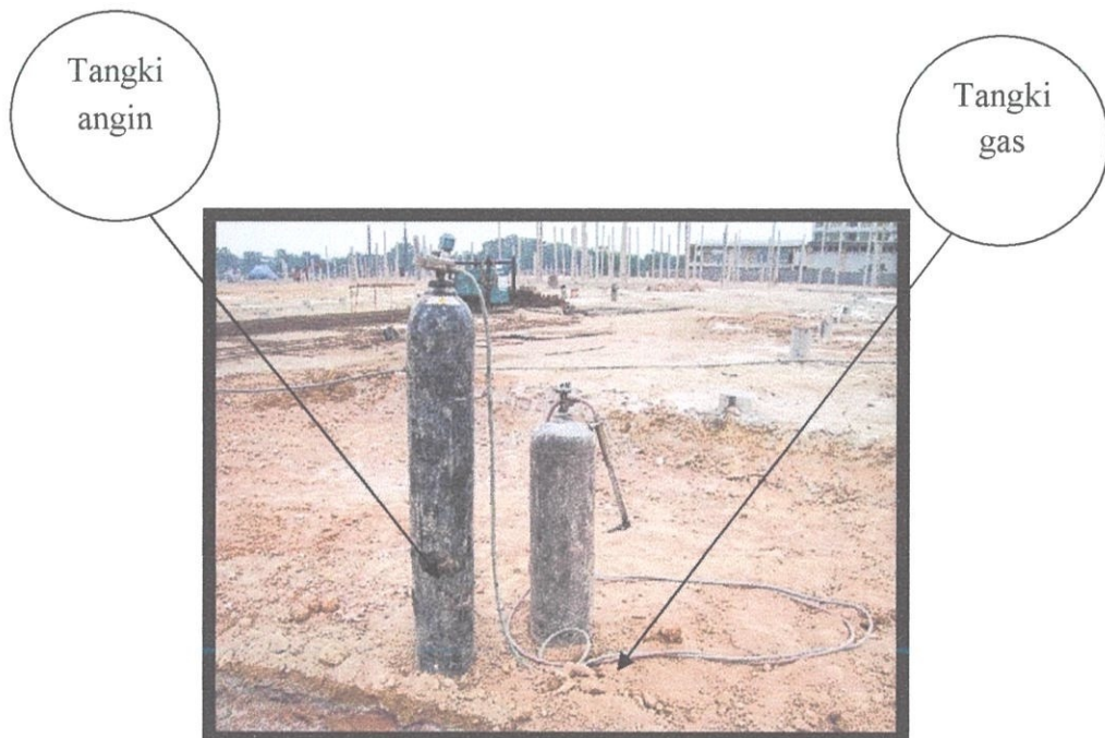
Gambarfoto 4.9: Tangki Gas (Oxy Tank)
