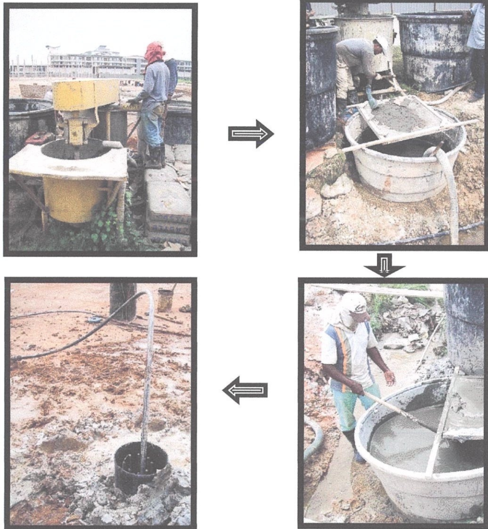
Gambarfoto 4.26 : Carta Proses Perekat (Grouting) 1
