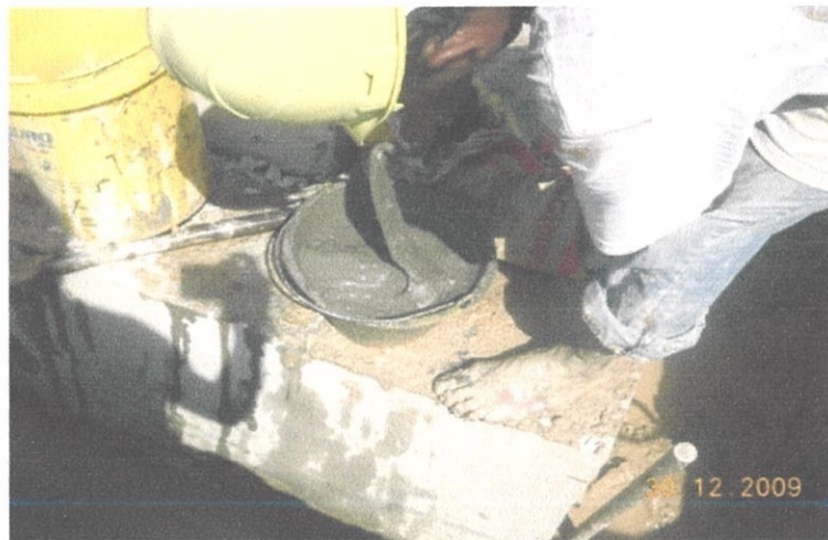
Gambarfoto 4.15: Pekerja membancuh Simen Sika Grout-215
