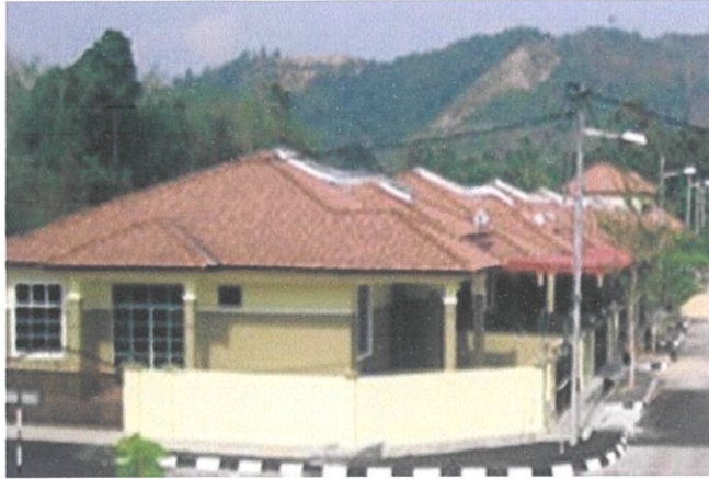
Photo 2.3 : Taman Jeniang Jaya ( Phase III )
