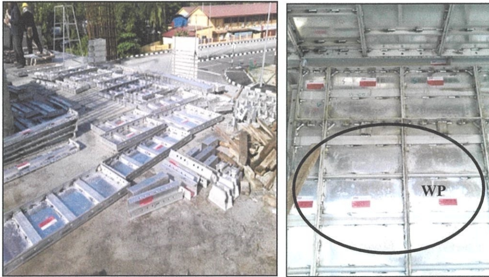
Photo 3.6: Wall Panel (WP), (WPF)
