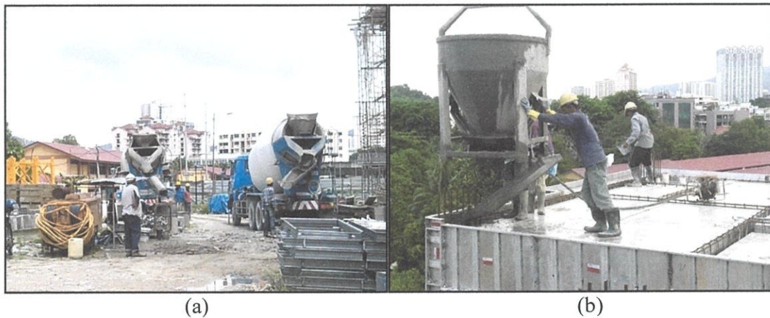
Photo 3.4 (a-b): Concreting Work at 4 th Floor Slab/ Beam (Unit 9 and Unit 10)
