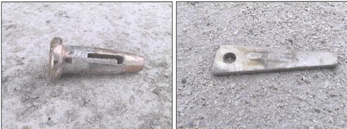
Photo 3.27: Steel Pin and Wedges
