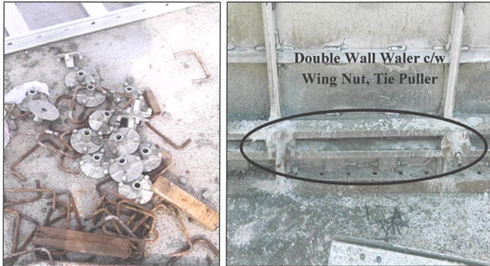
Photo 3.30: Double Wall Waler, Wing Nut and Tie Puller
