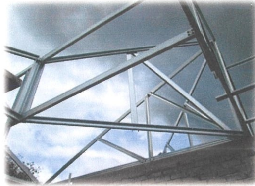
Figure 1.5: Half warren truss
