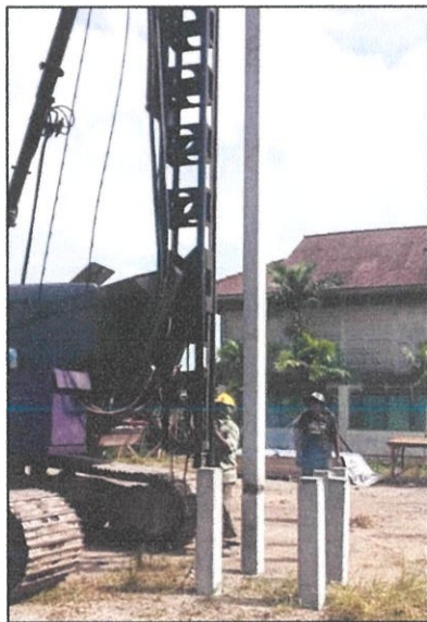
Photo 3.2.2 (a) : Pile driven process at site
