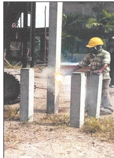
Photo 3.2.2(b) : Pile welding process
