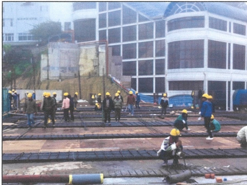
Photo 3.4: Photo before progress.
