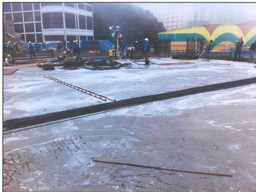
Photo 3.5: Photo after progress.
