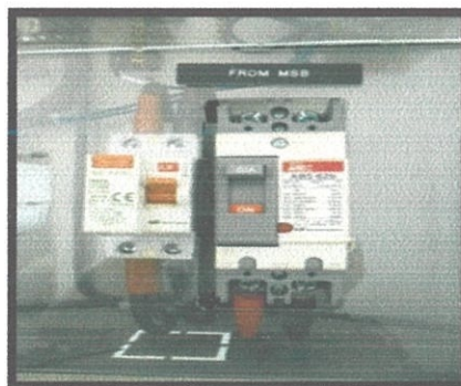
Diagram 3.2 : Residual Circuit Current Breaker
