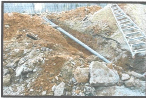
Diagram 3.1 : G.I. ducts laid inside the excavated soil
