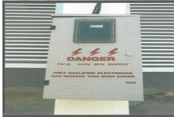
Diagram 3.1 : The electrical meter box
