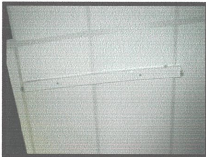
Diagram 3.3 : Fluorescent fitting c/w Daikon diffuser
