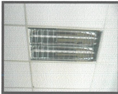
Diagram 3.3 : fluorescent fitting c/w aluminum parabolic louvers and mirror reflector
