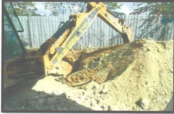
Diagram 3.1 : Excavating work for G.I. duct installation
