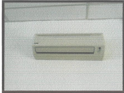
Diagram 3.6 : Unventilated split air-conditioner (evaporation unit)
