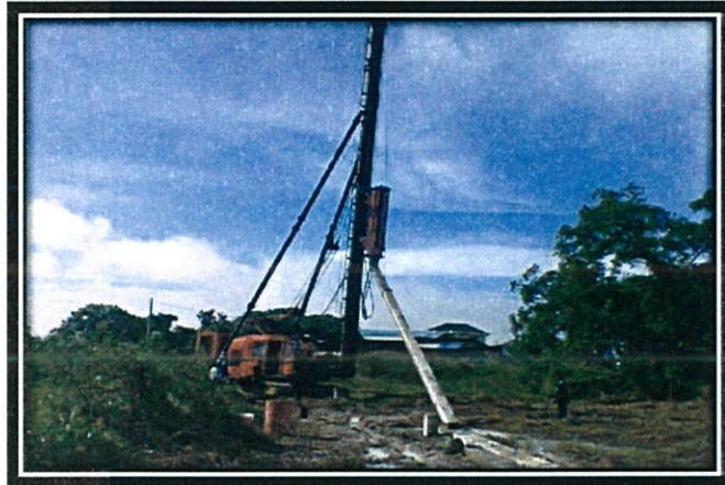
Picture 3.5: Pile lifting work to piling machine
