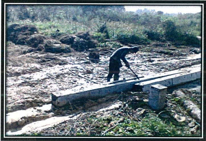
Picture 3.4: Marking pile rod work
