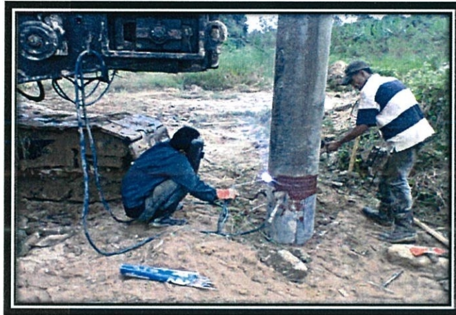
Picture 3.8: Connection on pile work
