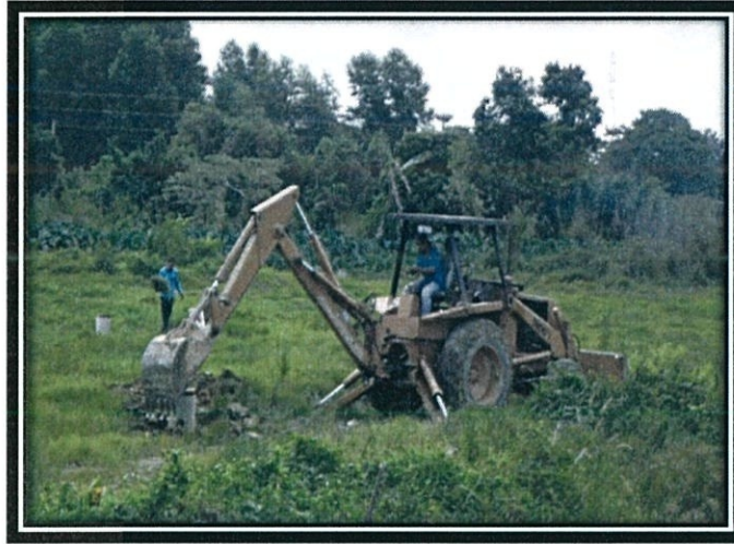
Picture 3.2: site clearance work
