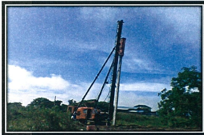
Picture 3.6: Blow the pile
