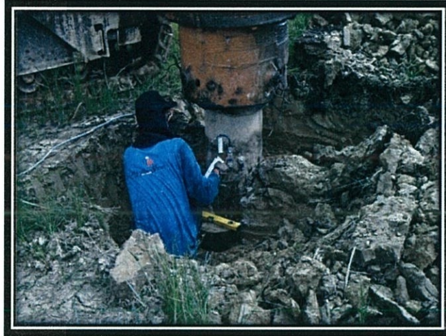
Picture 3.11: Wires of PDA devices put on the pile
