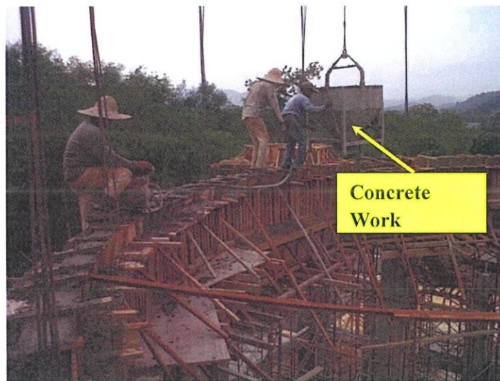
Photo 3.15 Concrete Works Grade 30 for Ring Beam
