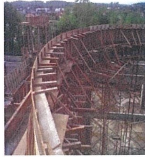
Photo 3.4 Formwork Installation
