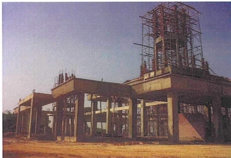
Photo 3.1 Construction of new mosque
