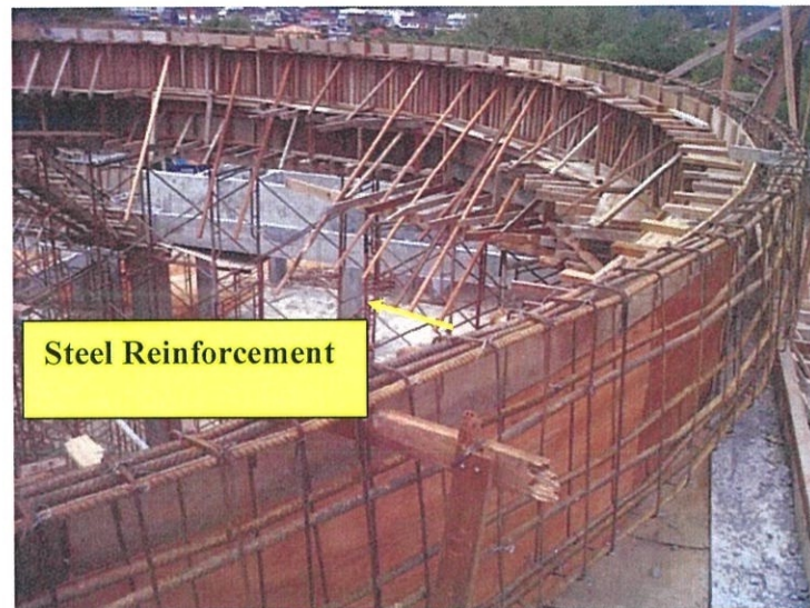
Photo 3.13 Installation of Steel Reinforcement at Ring Beam
