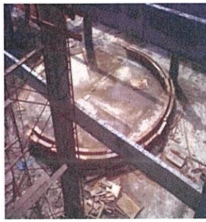
Photo 3.3 Circle Formwork
