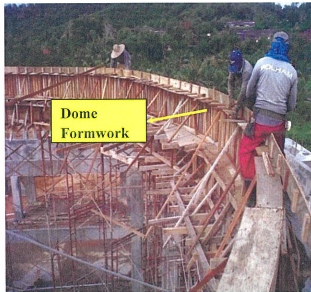
Photo 3.12 Installation of Internal Dome Formwork
