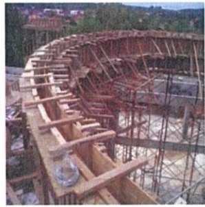
Photo 3.6 Lock Formwork
