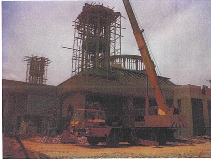
Photo 3.4.4 Crane that use during concrete work
