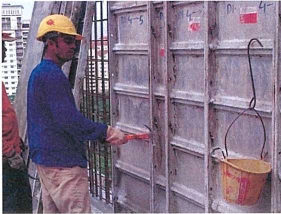
Figure 3.14: Example of Wall Panel installation
