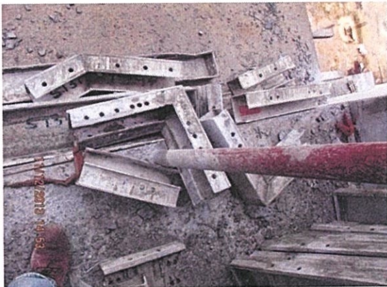
Figure 3.9: Examples of Slab Corner Joint
