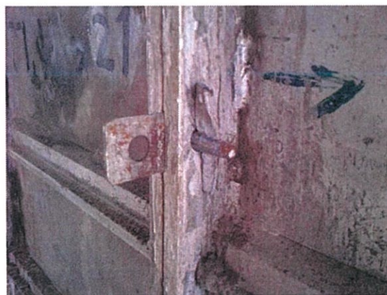
Figure 3.18: Examples Pin and Wedge position
