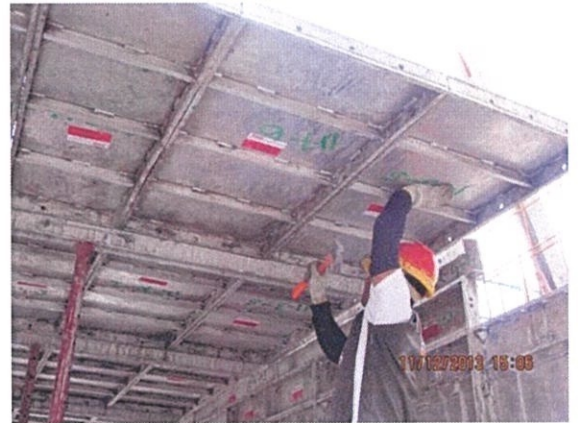
Figure 3.4: Example of Slab Panel
