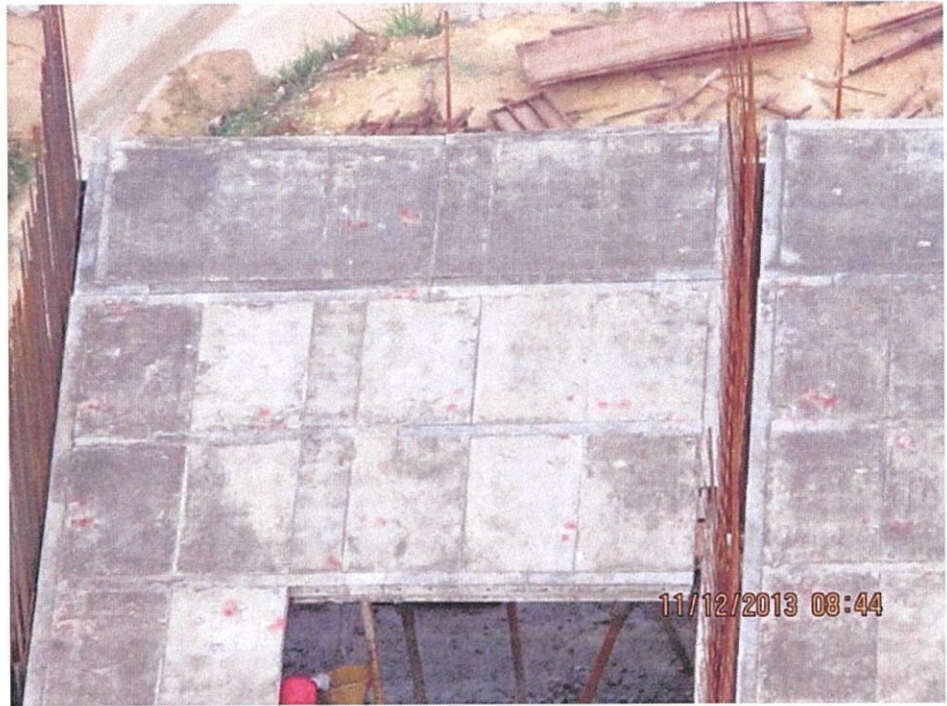
Figure 3.22: Slab Panel installation (cont'd)
