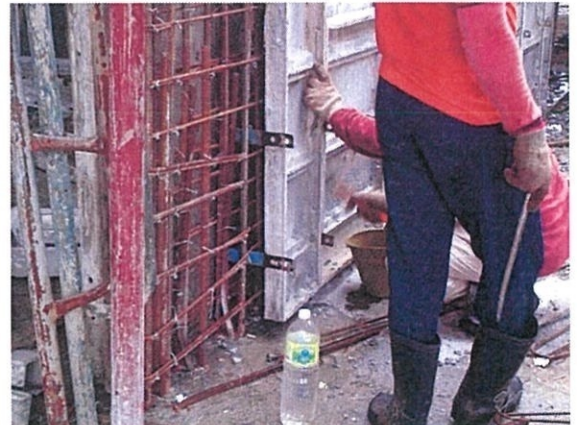
Figure 3.17: Installation Wedge and Pin
