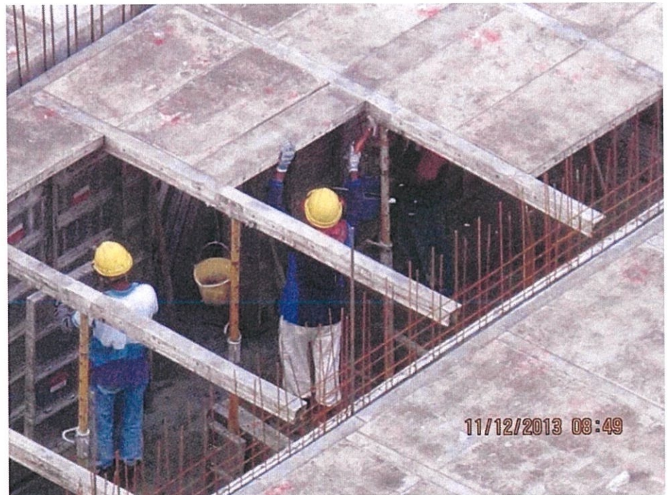
Figure 3.23: Installation of Slab Panel (cont'd)
