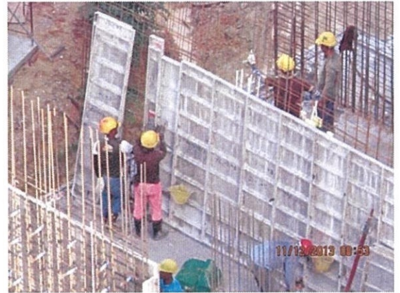
Figure 3.15: Wall Panel installation
