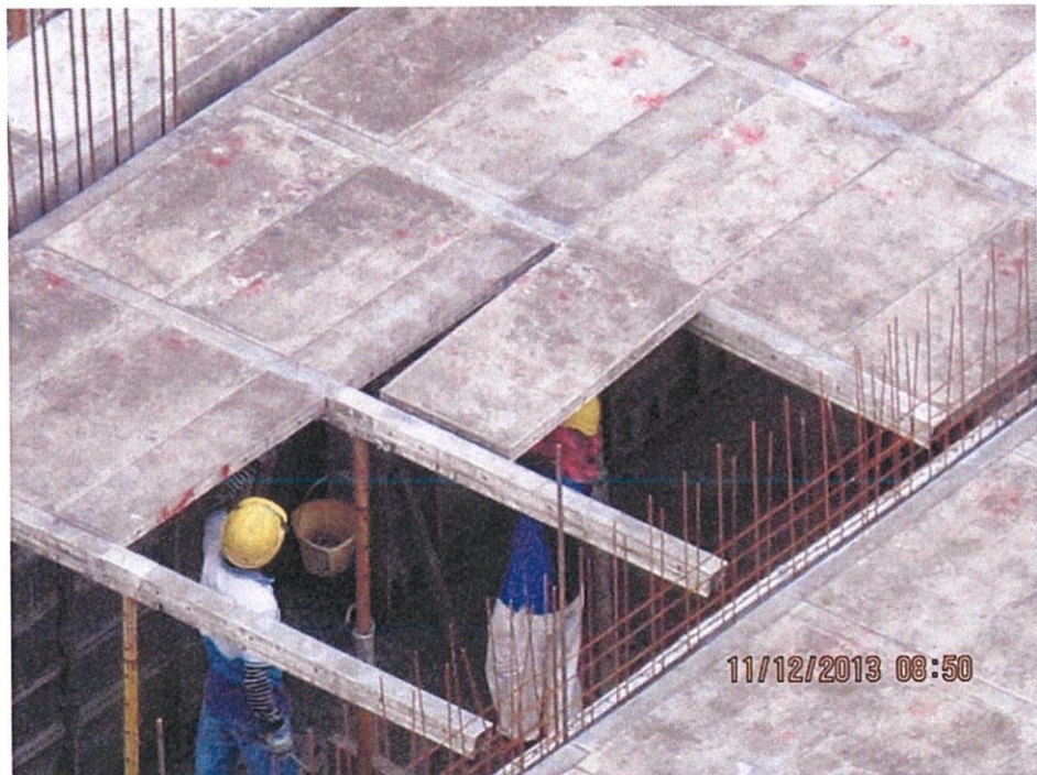
Figure 3.21: Installation of the Slab Panel
