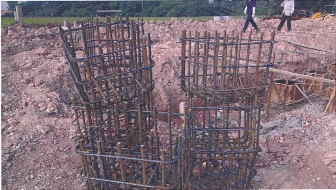
Photo 3.9 The pile cap reinforcement for 1 pile group.
