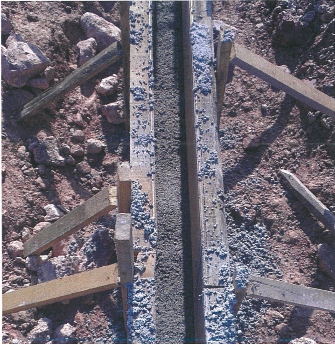
Photo 3.16 Lean concrete is poured before concreting.
