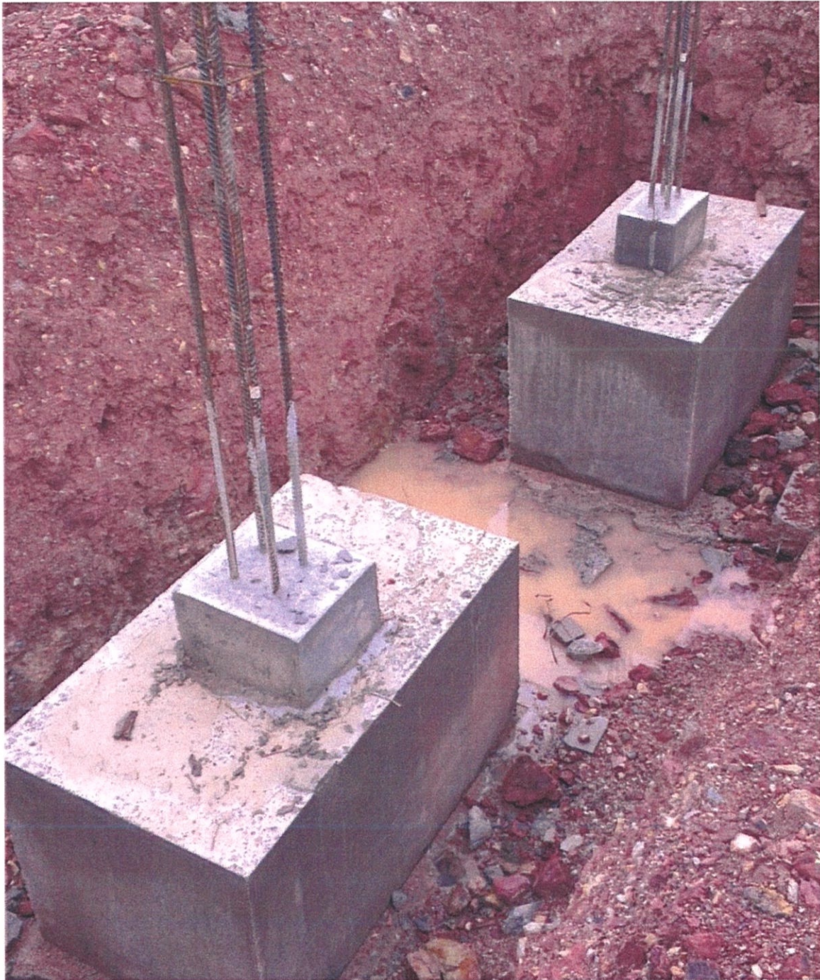
Photo 3.14 The column stump on the pile cap.
