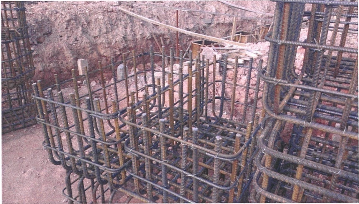
Photo 3.8 The pile reinforcement for 2 pile group.
