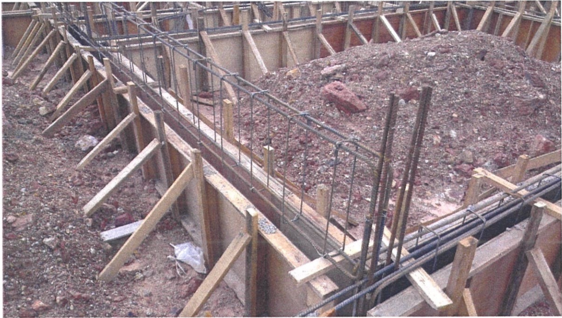
Photo 3.17 The reinforcement for ground beam.
