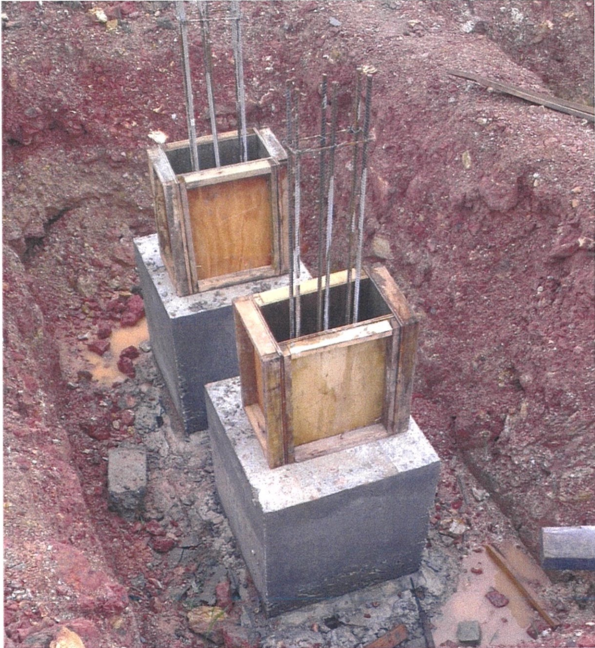
Photo 3.13 The formwork for column stump.
