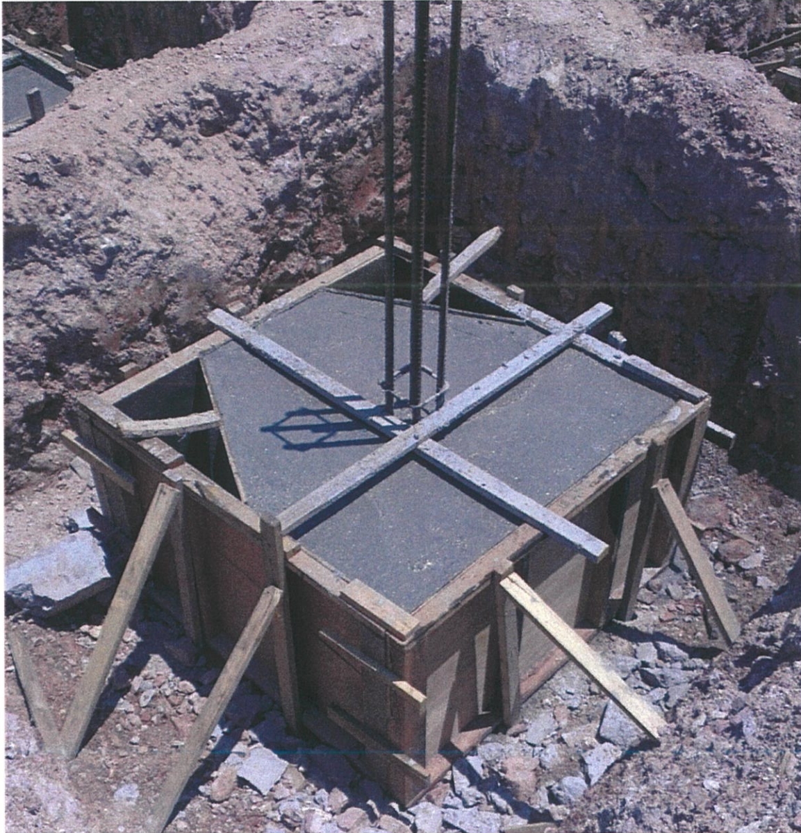
Photo 3.10 The concreted pile cap 3 pile group.
