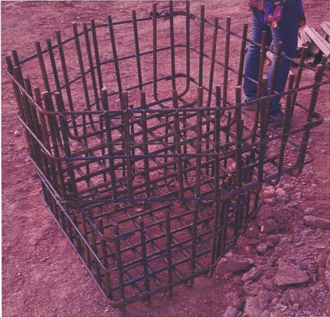
Photo 3.7 The pile cap reinforcement for 3 pile group.
