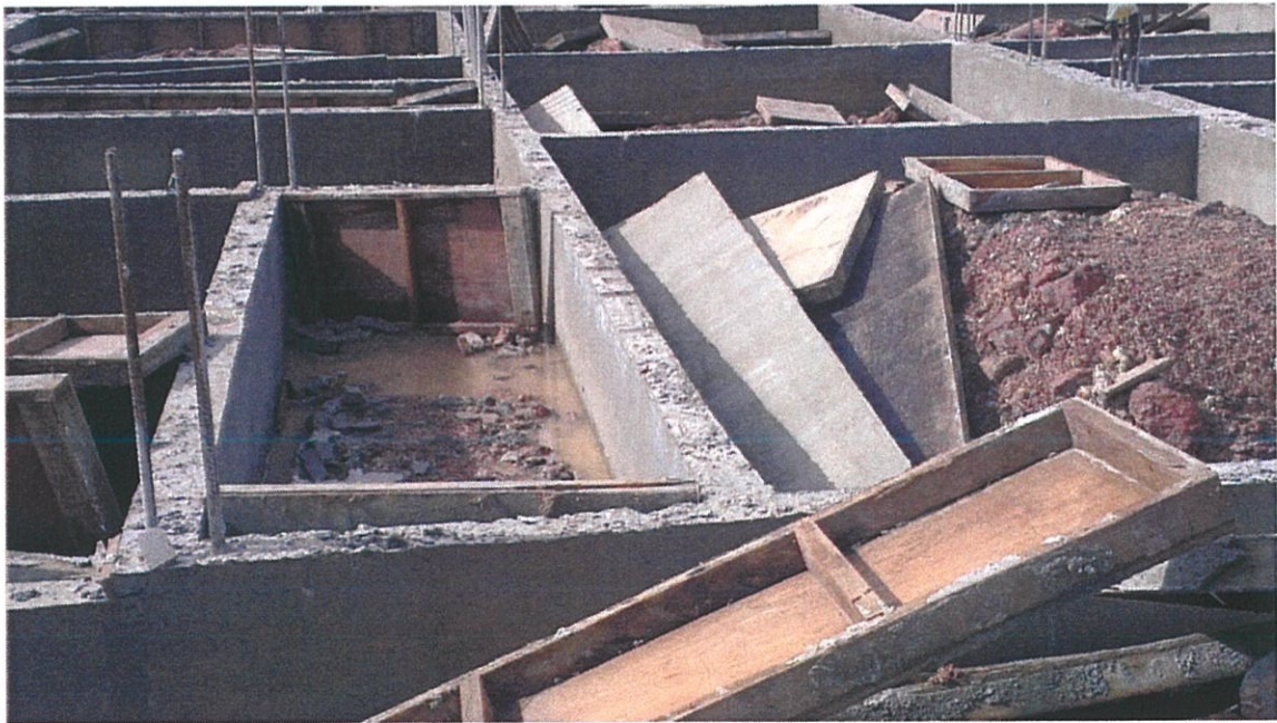
Photo 3.18 The ground beam.
