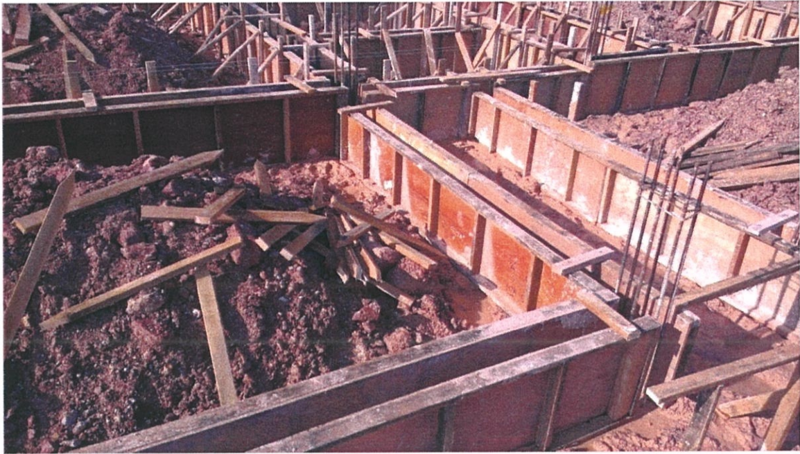
Photo 3.15 The formwork for ground beam.
