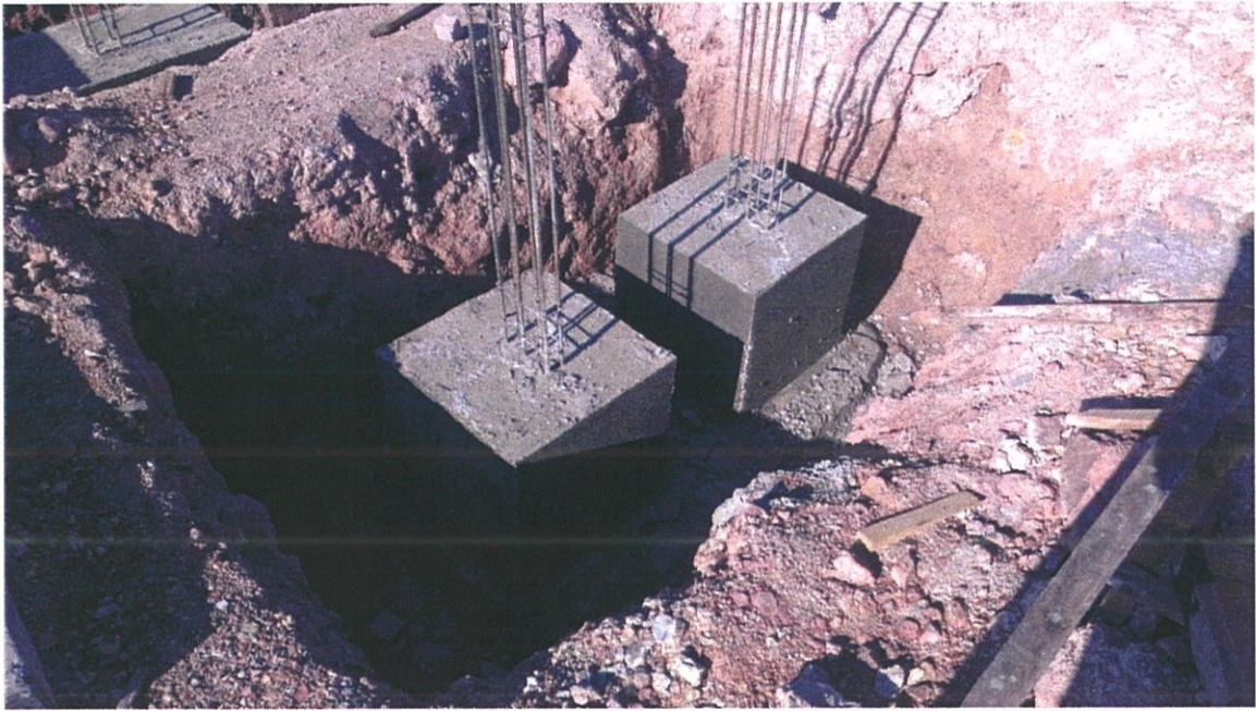
Photo 3.11 The pile cap for 1 pile group.
