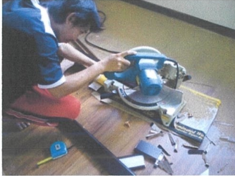
Rajah 4.2.7a– Memotong 'Skirting'
