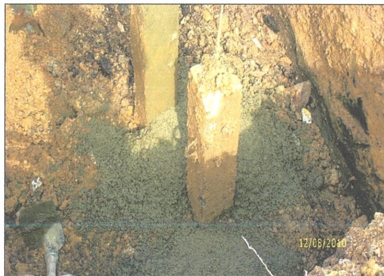
Rajah 4.5 Kerja Meletakkan Lapisan 'lean concrete'
