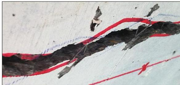
**Figure 6:** Steel fiber bridging the cracks of concrete
