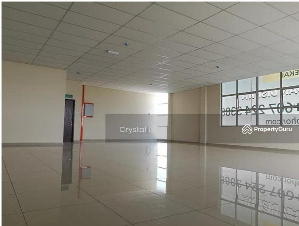
Figure 5.2.3 warehouse second floor
