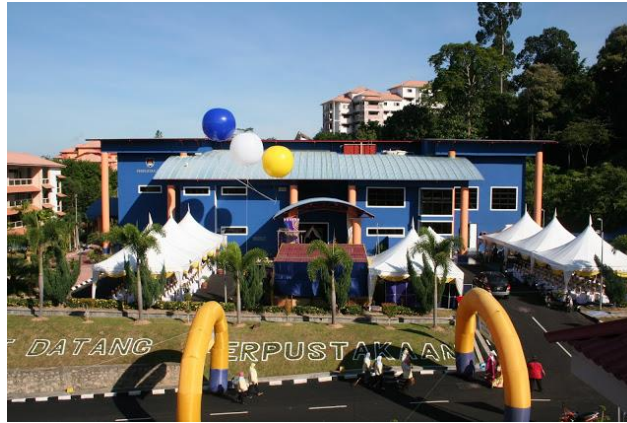
Figure 1.1 The building of Perpustakaan Tengku Anis
