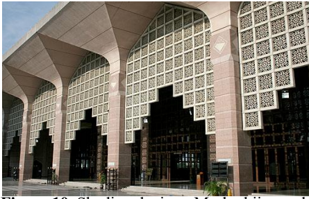
Figure 10. Shading devices, Mashrabiya and overhang roof of PM
