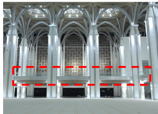
Figure 13. Daylighting penetrates the internal area of the main prayer hall, TMZAM, through the woven stainless steel mesh (mashrabiya), the skylight at the roof level and the air gap space at the dome
