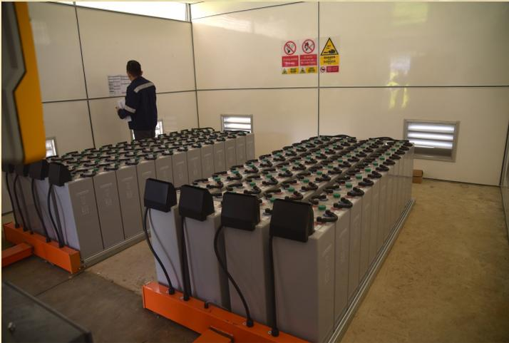
The 28.13kW standalone solar PV system is supplying electricity to 28 households of Iban community in the Rumah Panjang. The system was commissioned on November 2021 and designed to operate with 60% of the consumption supplied by battery and 40% by the solar PV.
