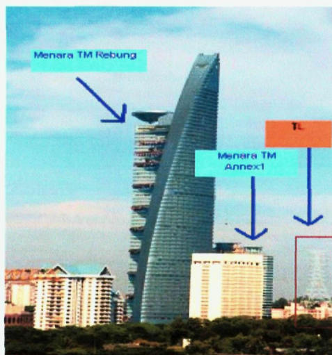
Figure 4: TL, Menara TM Rebung & Menara TM Annex 1
