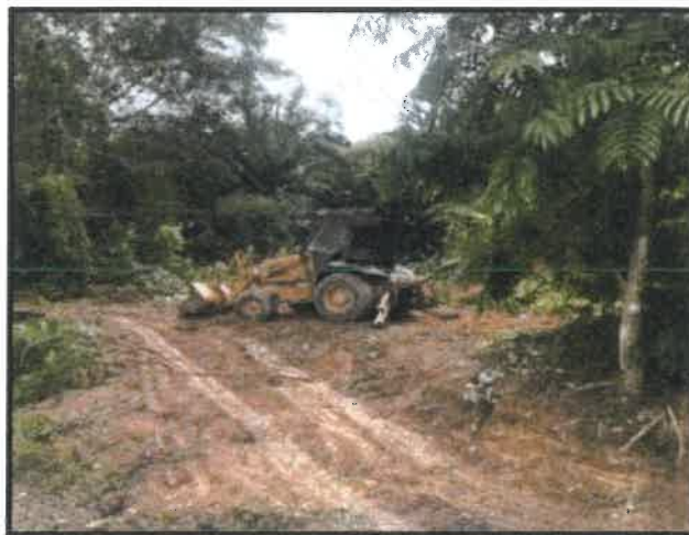
Figure 3.2 Site clearance work
