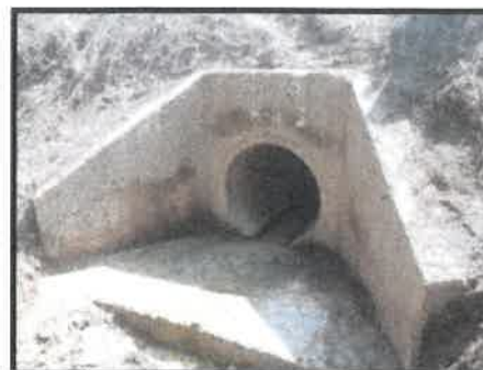
Figure 3.15 Pipe culvert
