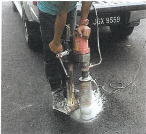
Figure 2.3 Drilling pavement for coring test
