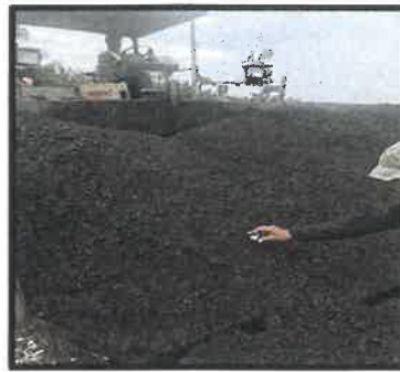
Figure 3.8 Measuring temperature of premix on paver machine
