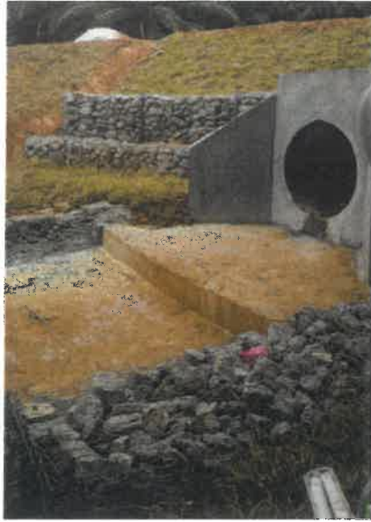
Figure 2.0 Slope treatment and culvert replacement
