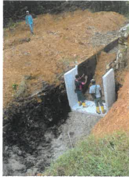
Figure 2.1 Drain replacement work
