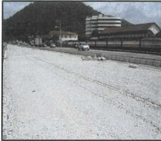
Figure 3.4 Crusher-run layer as roadbase
