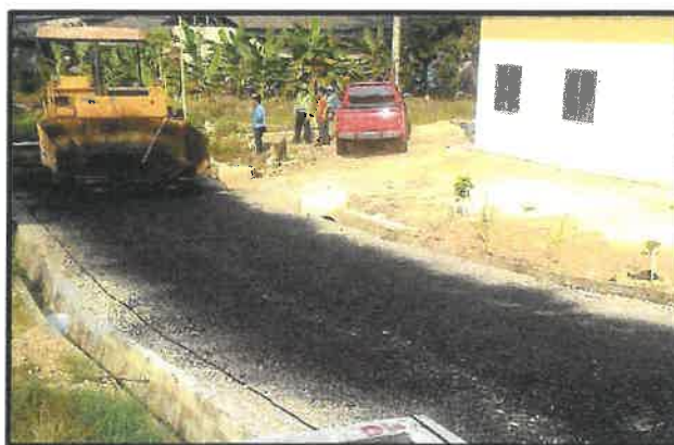
Figure 3.6 Roadbase sprayed with prime coat (bitumen emulsion SS1K)
