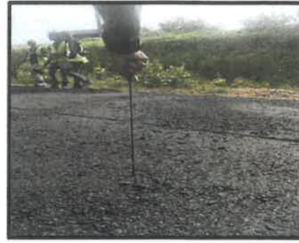
Figure 3.10 Dipping to determine laying thickness
