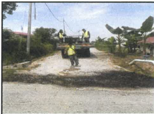
Figure 3.5 Spraying prime coat process
