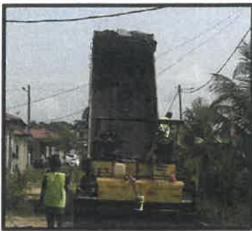
Figure 3.7 Transferring premix from truck into paver machine
