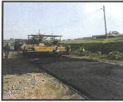
Figure 3.9 Laying premix using paver machine
