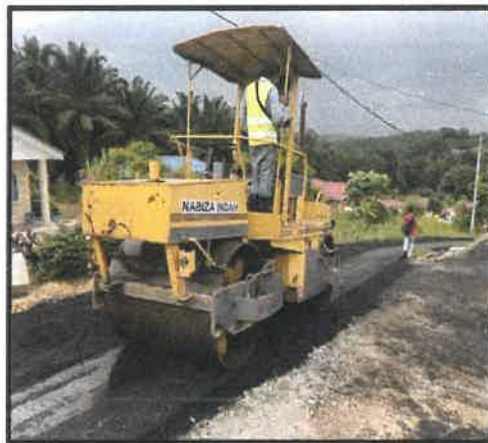
Figure 3.11 Tandem roller
