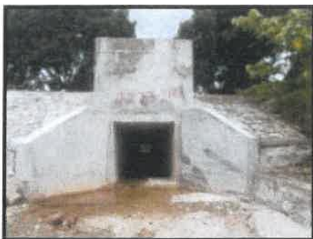
Figure 3.14 Box culvert
