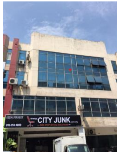
Figure 2.3 Front view of K&P Cove Consultancy
