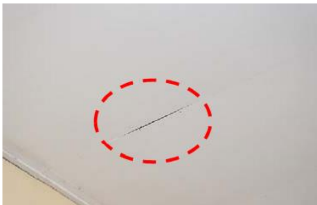
Figure 3.19 Separation gap between ceiling panel with other ceiling panel.
