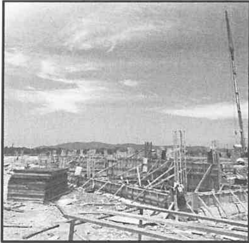
Ground Slab Formwork
