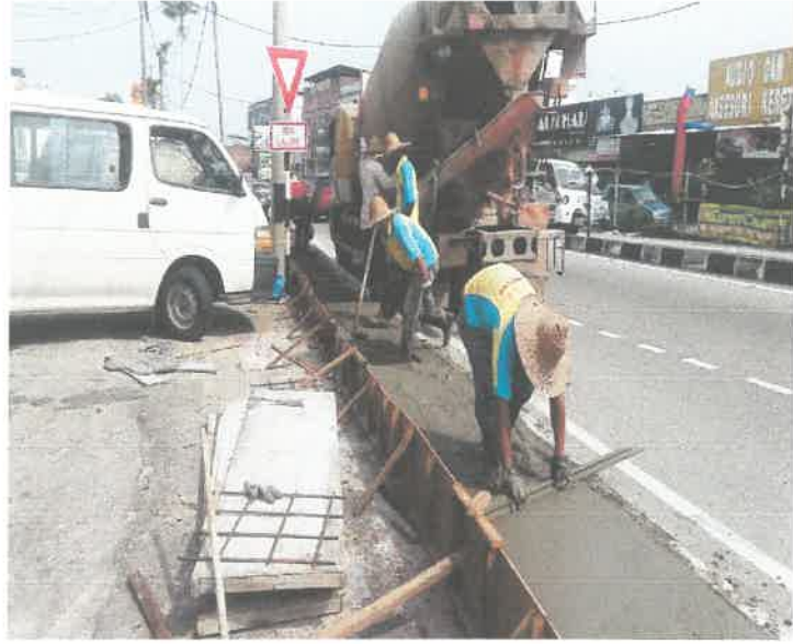
Figure 3.2.4.2 : Level and Flat the concrete
