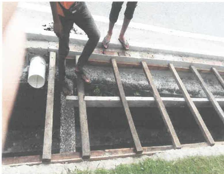
Figure 3.2.1.1 : Formwork of Drain
