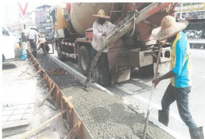
Figure 3.2.4.1 : Concrete poured on sheathing
