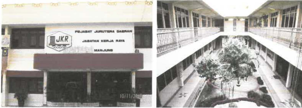
Figure 1.2.1 Jkr Manjung Office
