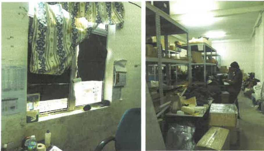
Figure 3.1.2 The Windows and The Room That Need To Be Renovate
