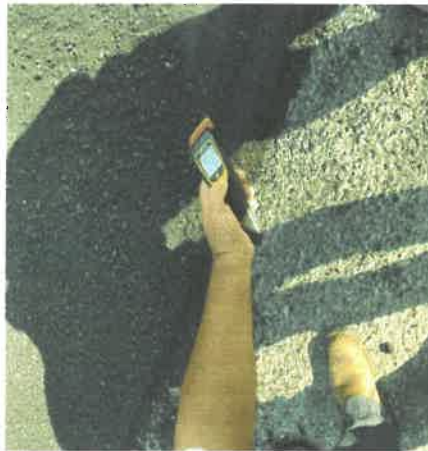
Figure 3.1.5 Checked Temperature at Paver and After Layer at Road Surface
