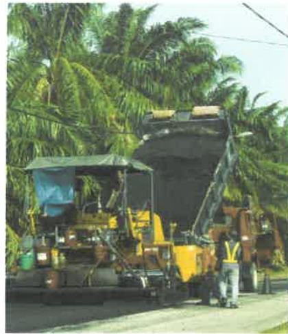
Figure 3.1.4 Tack Coat and Premix Transfer to Paver
