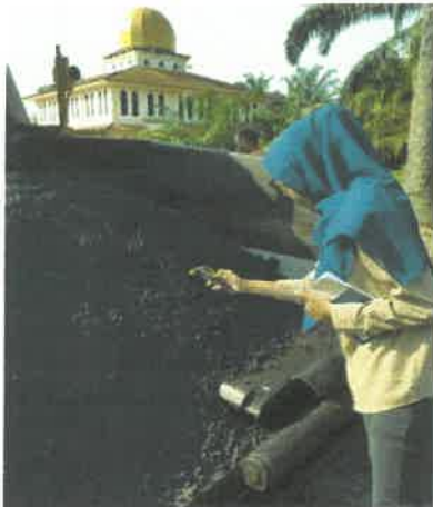
Figure 3.1.5 Checked Temperature at Paver and After Layer at Road Surface
