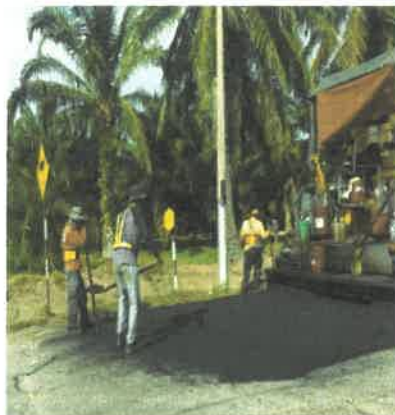
Figure 3.1.6 Hand casting Process and Paver machine
