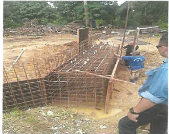
Figure 2.5 show the making of formwork of the abutment.
