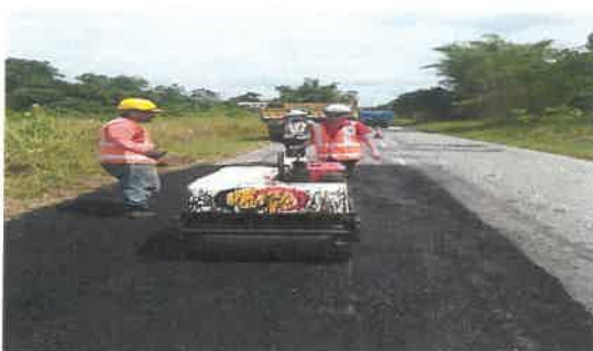
Figure 2.14 show the work of Shallow patching
