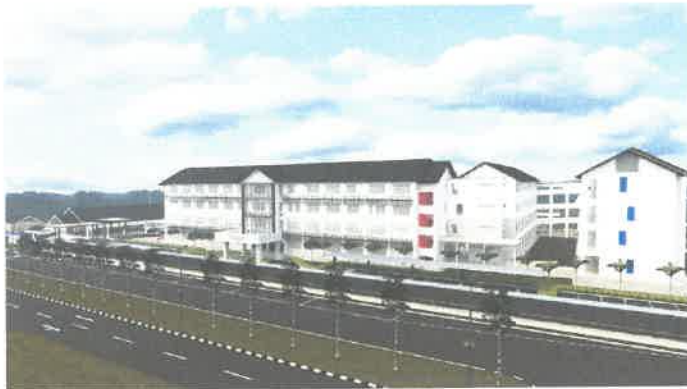
SMK Nilai Impian after finish construction (Figure 4.3)
