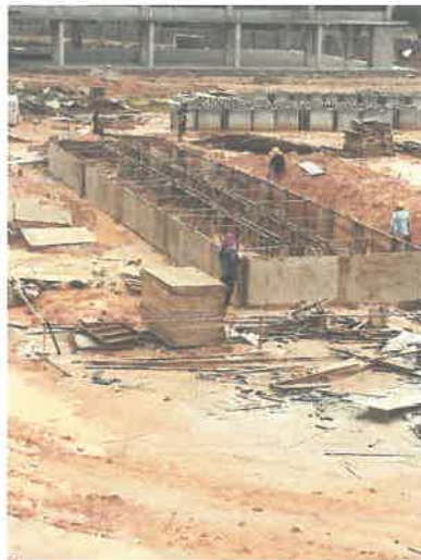
Installation of formworks and rebar for the beam of Astaka
