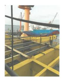
Figure 1.3: Example of primary beam attatch to secondary beam (I Beam)
