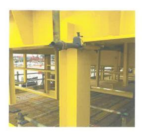
Figure 1.4: Pipe rack after final coat (yellow 550)
