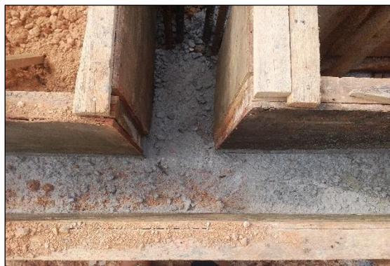
Figure 41: The Lean Concrete Use at Case Study
