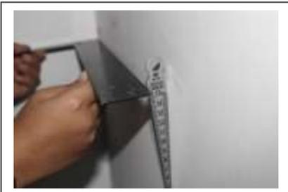
Wall squareness found misaligned and exceeded the tolerance of 4mm over 300mm (more than 15.0mm)
