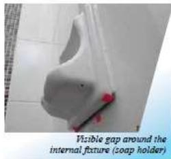
Figure 2. 22 : Defects on fixture
