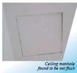
Figure 2. 19 : Defects on ceiling
