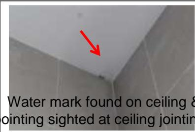
Water mark found on ceiling & pointing sighted at ceiling jointing
