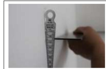
Wall squareness found misaligned and exceeded the tolerance of 4mm over 300mm (approximately 13.9mm)
