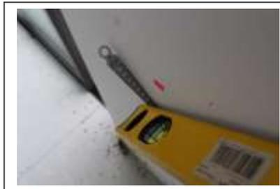
Wall found uneven and exceeded the tolerance of 3mm over 1.2m
