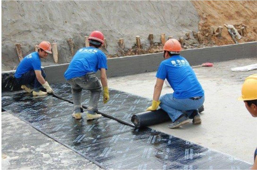
Figure 2.13 Bituminous membrane waterproofing
