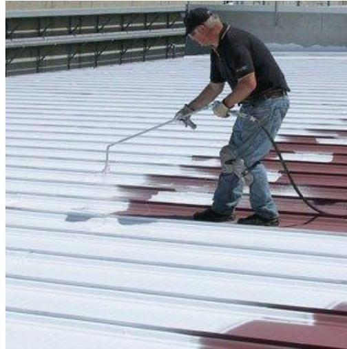
Figure 2.11 Liquid waterproofing membrane
