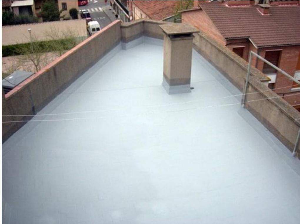
Figure 2.14 Polyurethane Liquid Membrane
