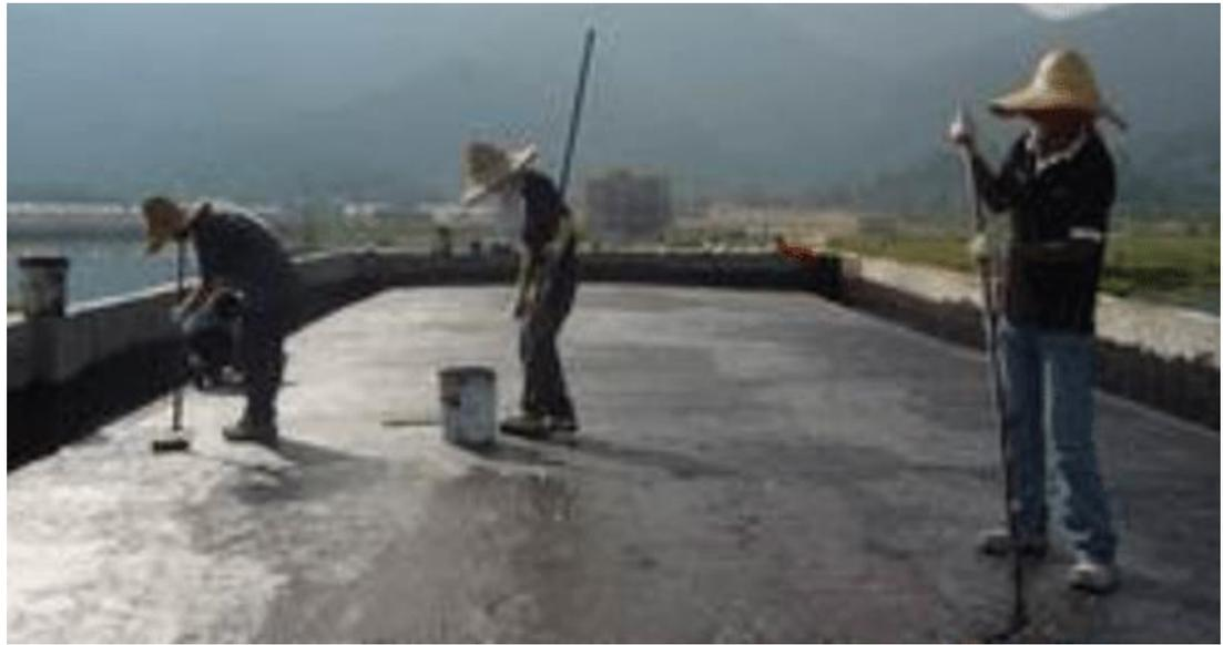
Figure 2.12 Bituminous coating waterproofing
