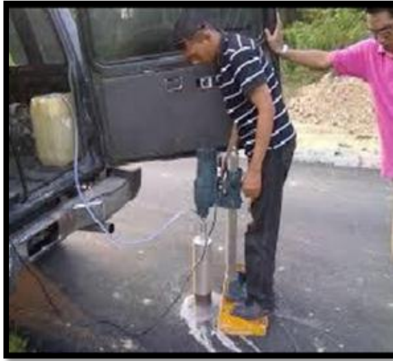
Figure 3.4 : The worker was drill the premix surface
