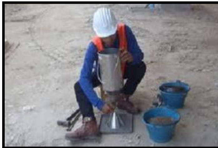
Figure 3.2 : The worker put the soil into the Dynamic Cone Penetration Test
