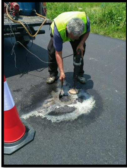
Figure 4.24 : The new premix was put into the hole.
