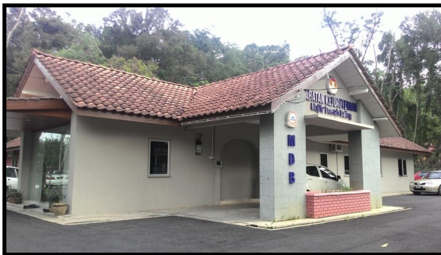
Figure 2.7 : Office of Engineering Department
