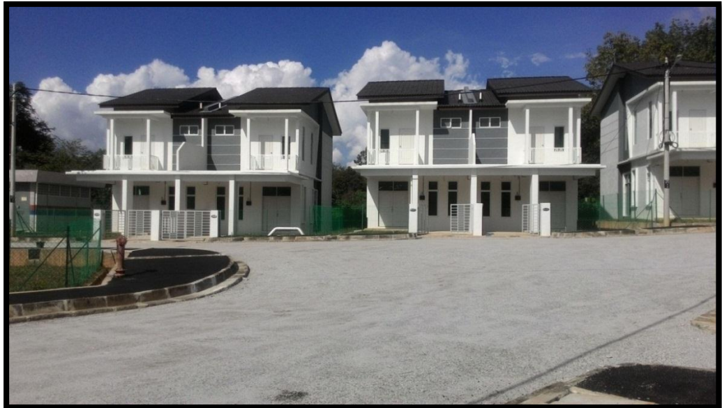
Figure 4.3 : Site of Case Study
