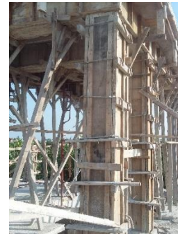
Figure 3.4.4: Formwork of column
