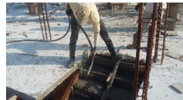
3.5.5: vibrating process
