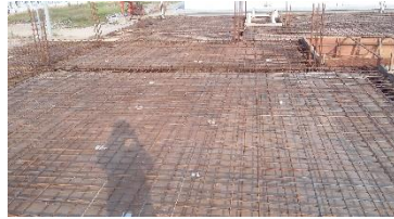
Figure 3.7.1: installation BRC steel
