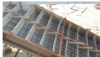
3.5.2: staircase formwork
