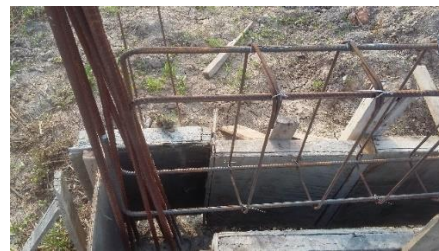
Figure 3.2.3: steel bar and link in ground beam
