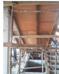
3.5.3: Soffit and struts of staircase formwork
