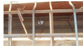
Figure 3.6.2 : spacer block
