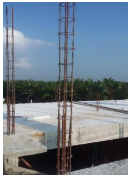
Figure 3.4.3: Reinforcement bars and link
