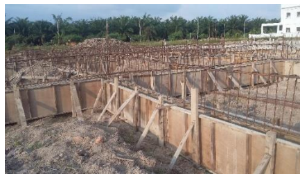
Figure 3.2.2: formwork
