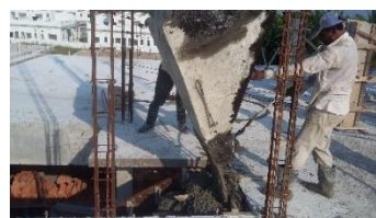
3.5.4: concreting work of staircase
