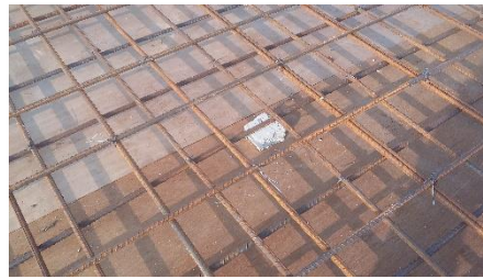
Figure 3.3.2.3: spacer block
