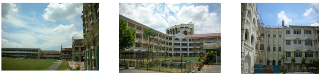
Figure 14: Insensitive additions to historic buildings at ACS and St. Michael's, Ipoh
