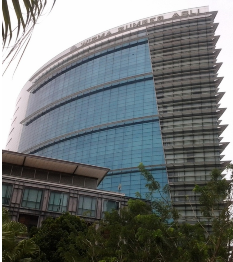
Figure 1.0 Natural Resources and Environment building
