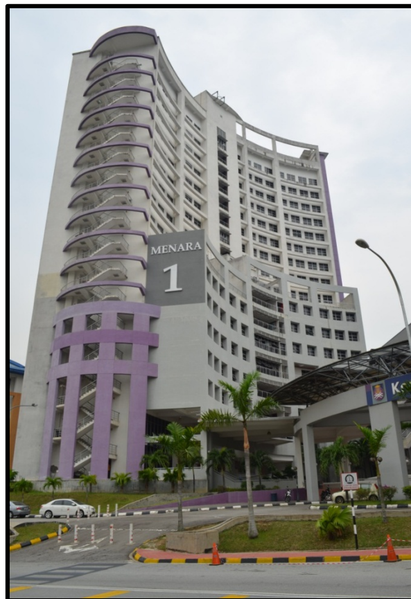
Figure 1.0: Science & Technology Tower from front view
