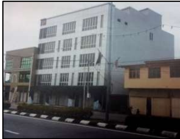
Photo 3.1 3 Units of 4 Storey Shop
