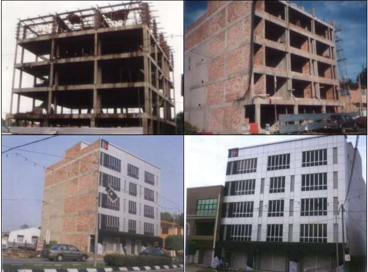
Photo 3.4 Case Study Building During Construction
